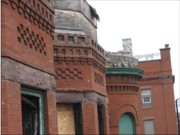
Figure 21 Note exposed Parapet wood work and brick back up on Street side
