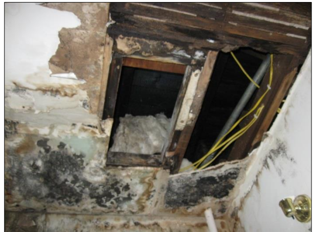
Figure 10 Roof leak and mold condition
