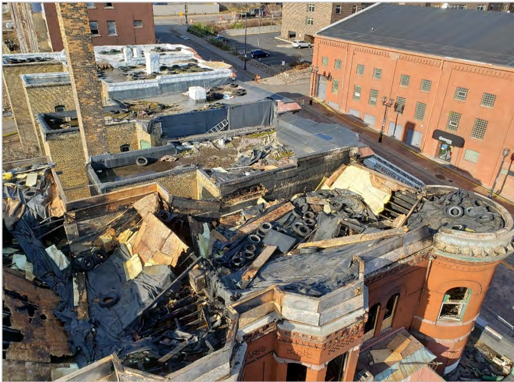
Photo 8: Collapsed fire damaged roofs of Pastoret Building westerly and easterly modules in foreground and roofs of modules bordering/running up 2 nd Avenue East beyond.
