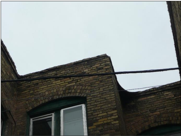
Figure 31 Brick parapet on rear of building in need of repair
