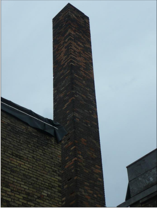
Figure 29 Brick chimney needs to be tuck-pointed
