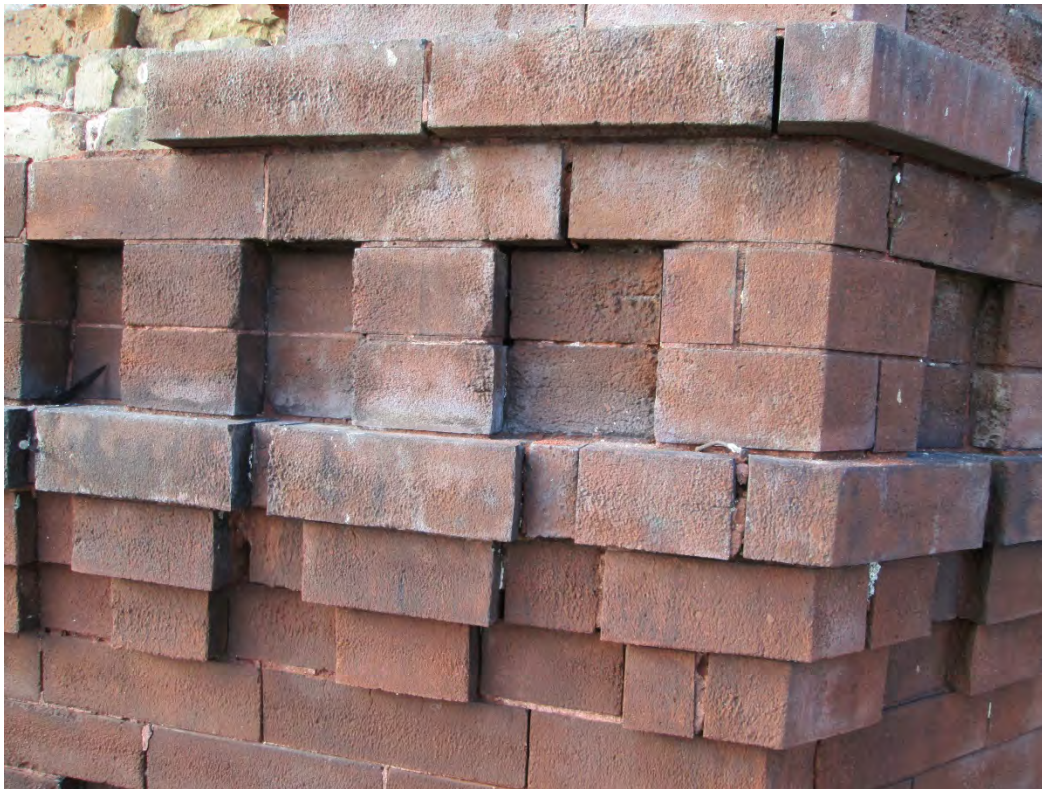
Photo 18: Close up, right end of previous photo (upper wall, south elevation). Note substantial efflorescence, face pitting in brick (potentially fire damage) and deteriorated pointing mortar.
