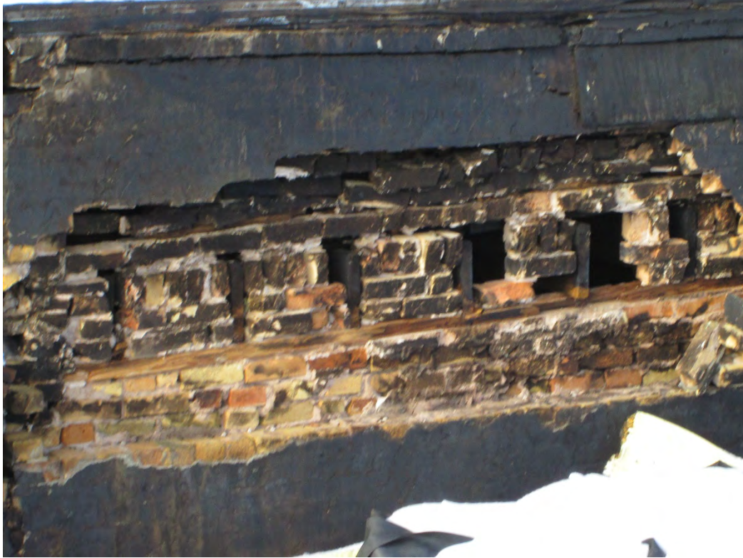
Photo 25: Party wall between east southerly Pastoret module and module to north. Some apparent fire damage to north module roof joist ends. Unknown (due to access limitations) if joists have suffered fire damage which is compromising structural stability of north module roof.
