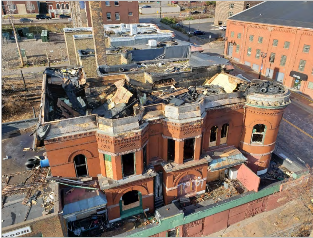
Photo 1: Southerly (1 st Street) Elevation of Pastoret Building. Westerly module is on left and easterly module is on right. Roof region and majority of window openings on both modules are open to the elements.
