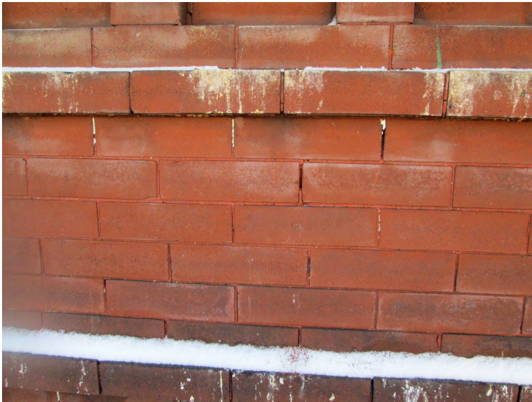
Photo 12: Typical exterior brick masonry wall pointing mortar condition at mid-wall regions, southern elevation shown.
