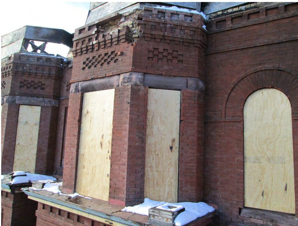
Photo 16: Looking slight west, upper region, south elevation. Substantial brick loss, loose bricks/displaced bricks.
