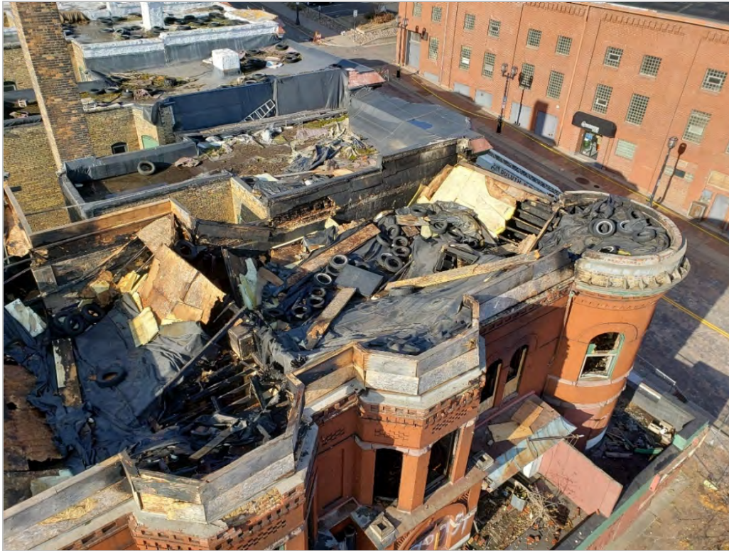
Photo 5: Fire destroyed and collapsed roof system of Pastoret Building easterly module.
