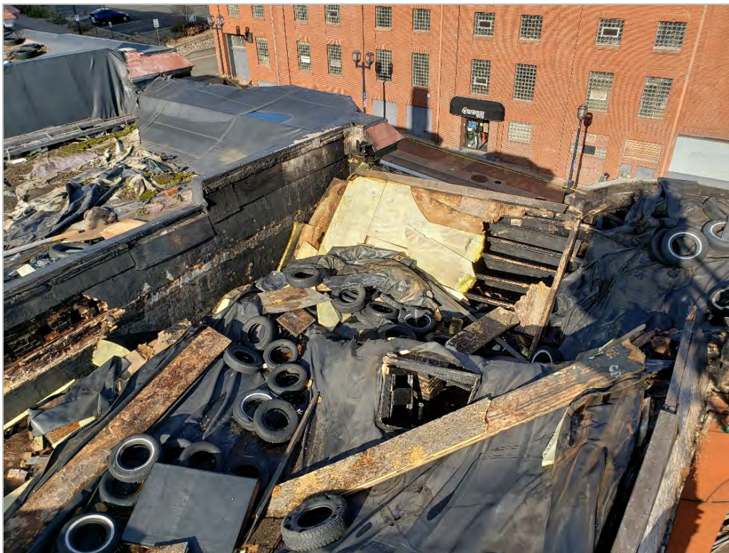
Photo 6: Close up view of fire destroyed and collapsed roof system of Pastoret Building easterly module.
