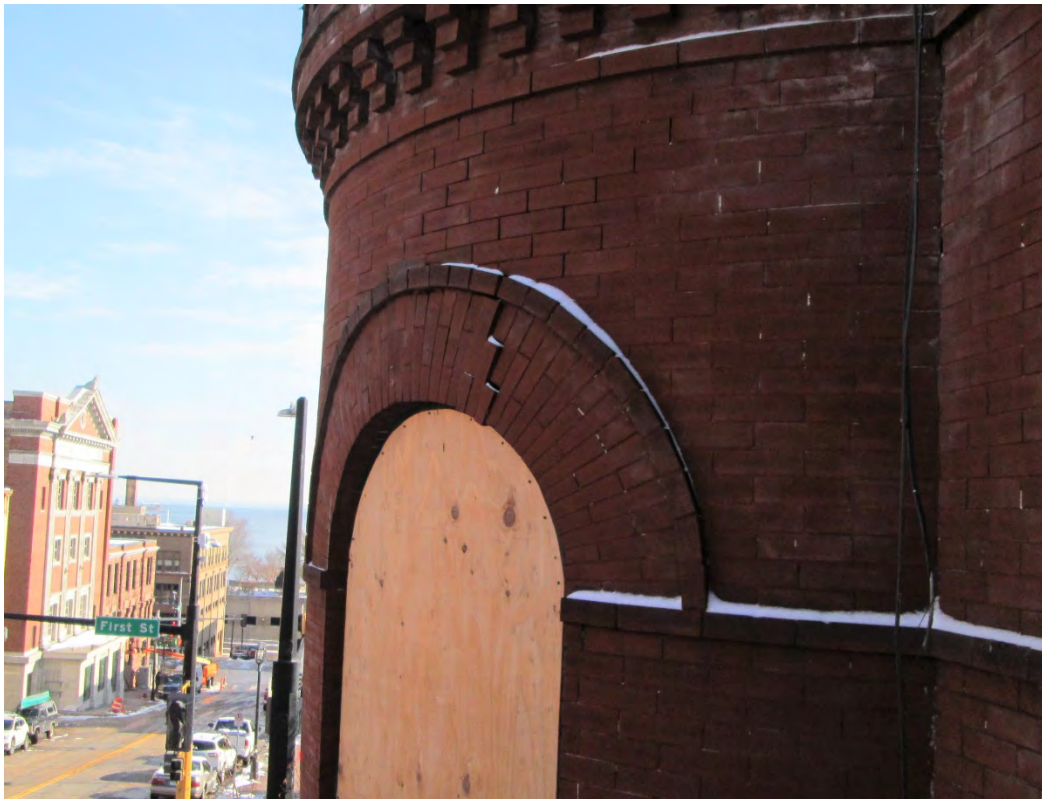
Photo 20: Southeast corner turret, looking south. Widened brick end joints and failing brick in window header arch may indicate larger movement/instability.
