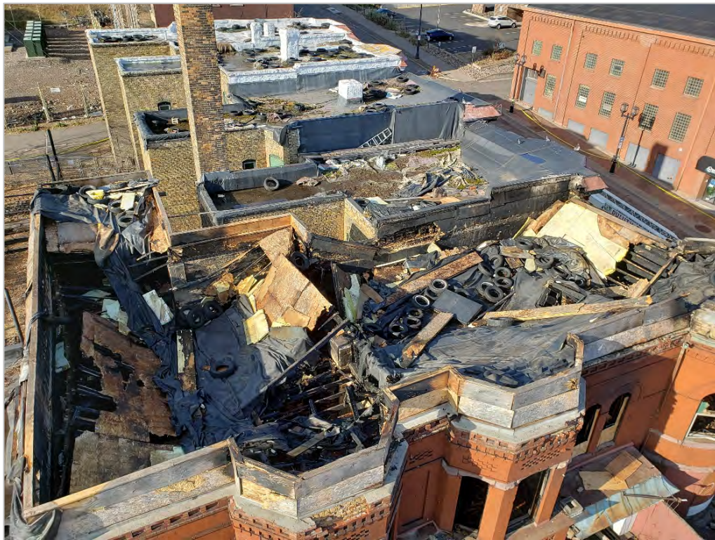
Photo 2: Fire destroyed and collapsed roof systems of Pastoret Building westerly (left side) and easterly (right side) modules.
