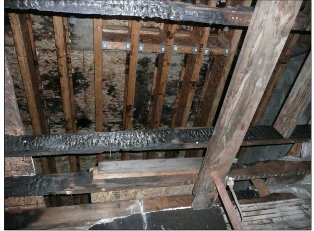
Figure 34 Fire damaged ceiling joists, temporary wood I-joist roof over fire damaged portion of the building
