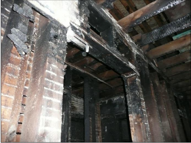
Figure 33 Fire damaged ceiling joists and wall framing
