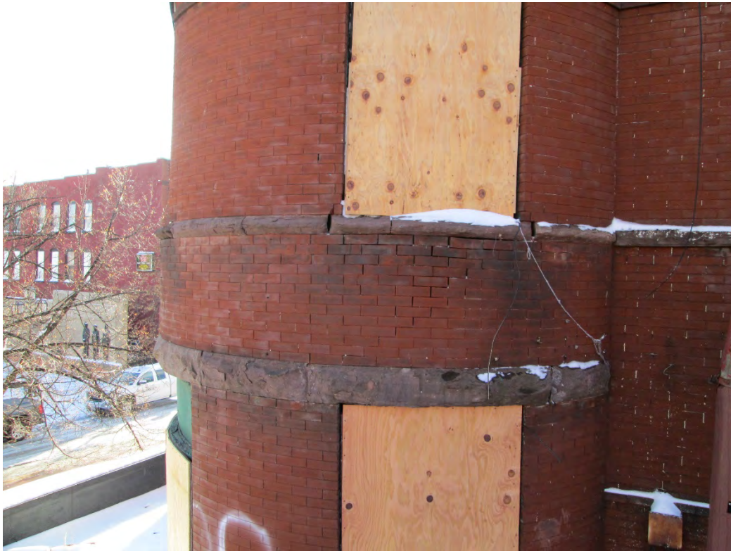
Photo 21: Region towards base of window in previous photo. Widened brick end gaps here also indicate potential global movement in circumference brick.
