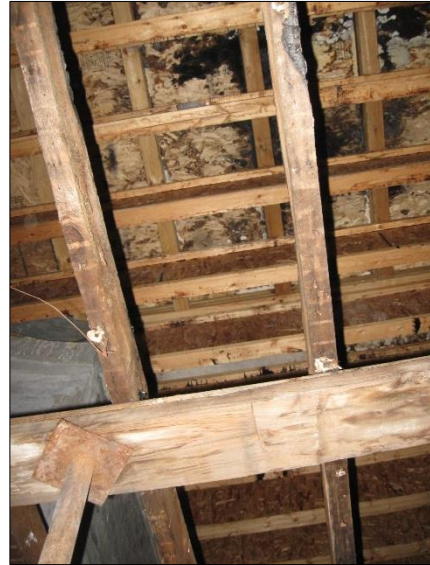
Figure 22 Black areas of temporary roof framing showing water intrusion and rot above burn area on Street side
