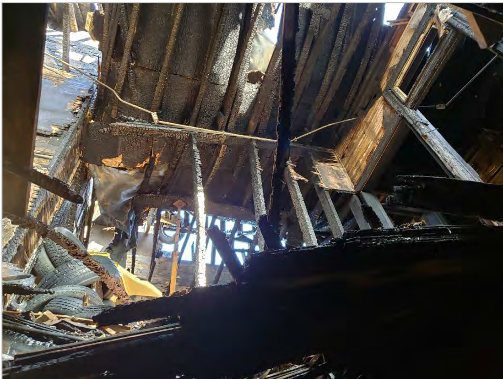
Photo 10: Looking Easterly from location shown in Photo 9 (Level 2, Pastoret Building westerly module). Ceiling above is burnt out/ collapsing onto Level 3 floor beneath. Large openings through collapsed roof which has fallen onto Level 3 can be seen.
