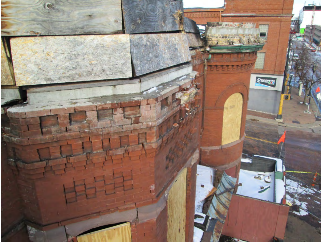
Photo 15: Looking east, upper region, south elevation, brick displacement/loose brick, significant efflorescence and loss of pointing mortar.
