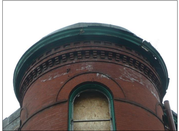
Figure 24 Loose brick at window arch, brick needs to be tuck-pointed
