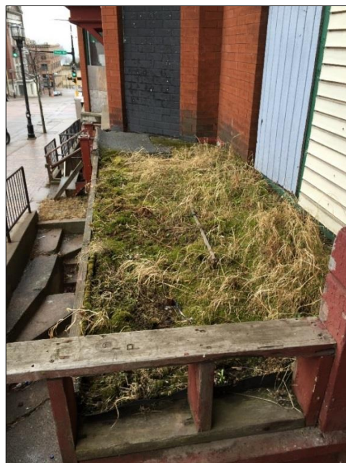
Figure 40 Vegetation growing on low roof, deteriorated roof structure below
