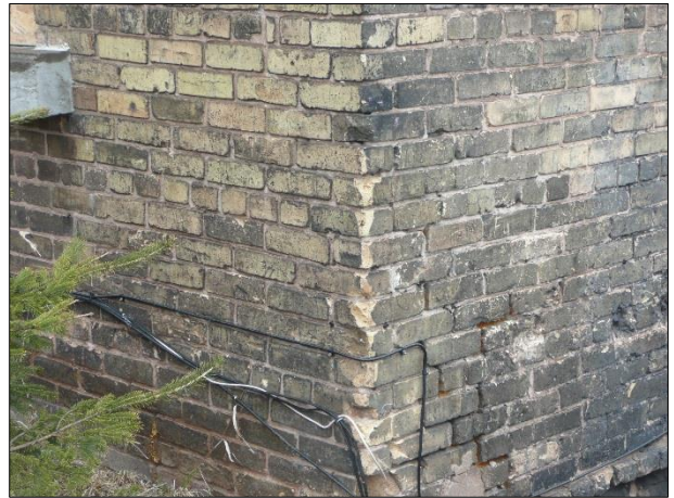
Figure 32 Damaged brick on rear of Pastoret building, brick needs to be tuck-pointed
