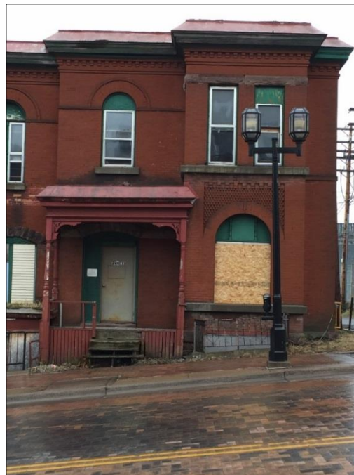
Figure 38 Entry stairs need to be replaced. Wrought iron railing needs to be repaired or replaced.
