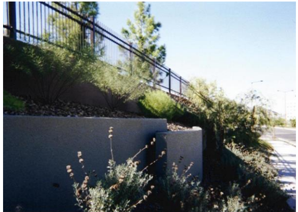
Figure 50-26.4-B: Retaining wall terracing and articulation
