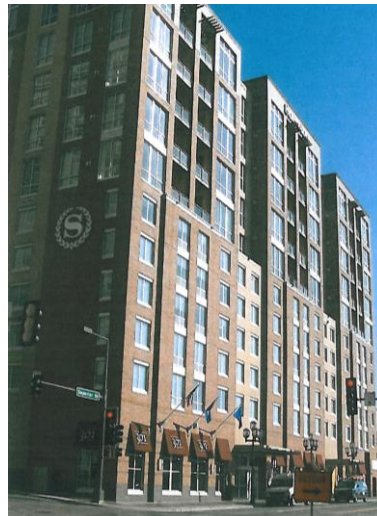
Example of Corridor Building III
