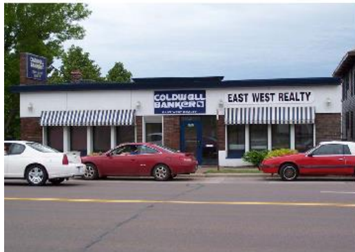
Example of Corridor Building I
