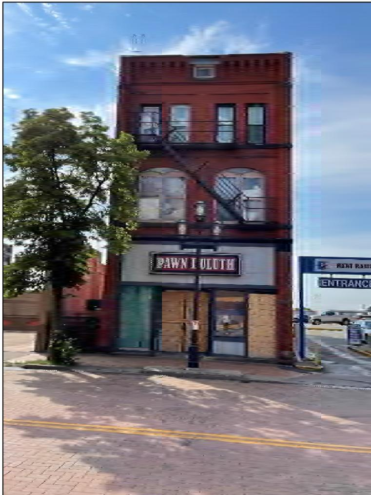
*Photograph 22: View of 126 E. 1<sup>st</sup> Street New stairways and fire escapes should not be added to the façade of historic structures within the historic district.*
