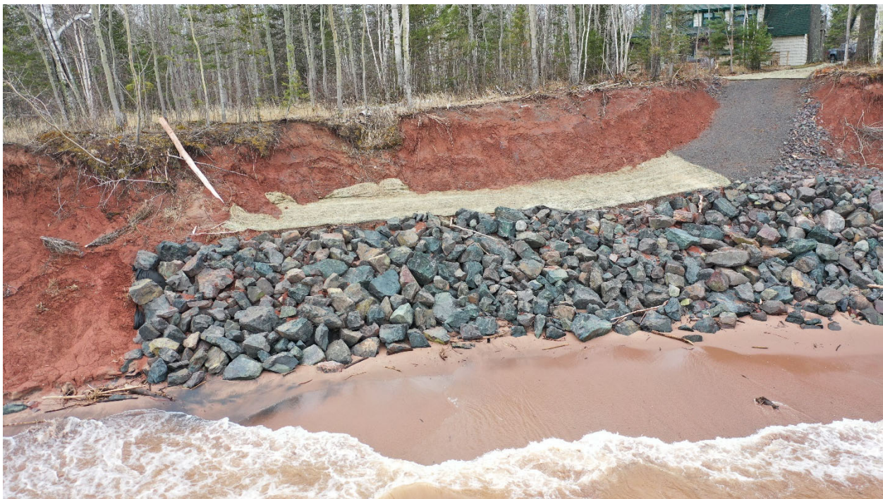
Figure 2. Heavy Riprap that was improperly installed by end dumping.
