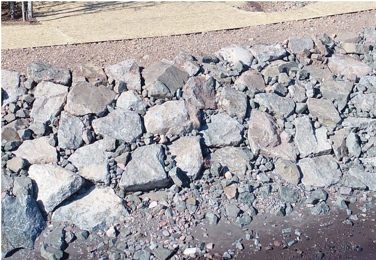
Figure 1. Properly constructed revetment
