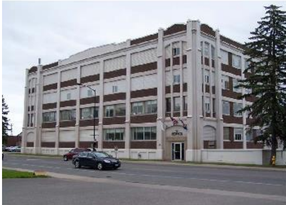
Example of Main Street Building III
