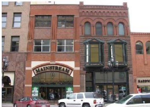
Example of Main Street Building III
