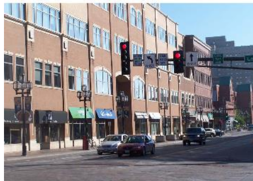
Example of Main Street Building III
