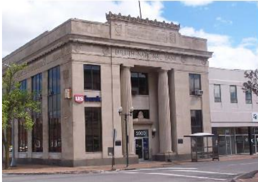
Example of Corridor Building II
