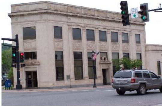
Example of Corridor Building II
