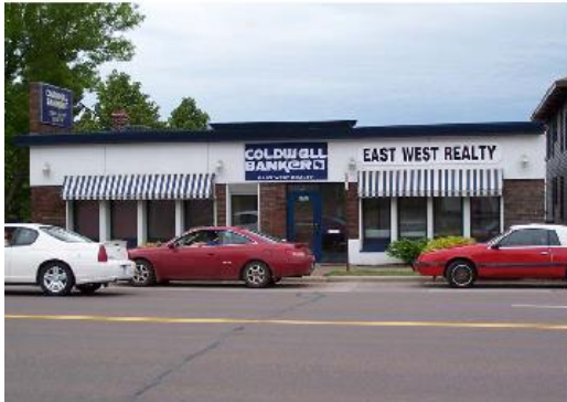
Example of Corridor Building I
