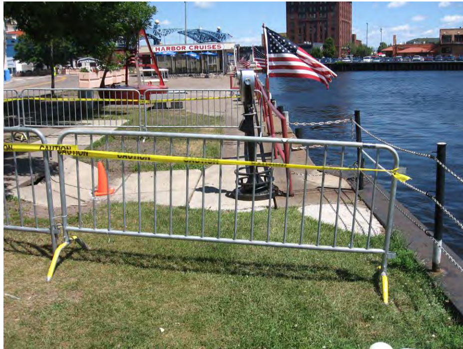
Figure 8. Sinkholes forming behind the DECC
