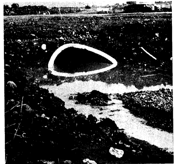
Soil erosion during the construction of K-Mart in 1975.
