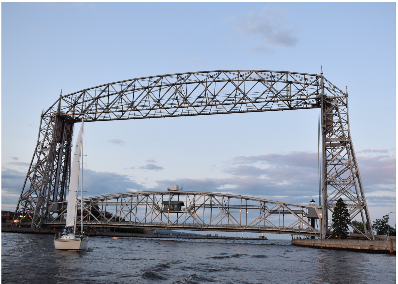
Aerial Lift Bridge
