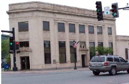
Example of Corridor Building II
