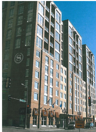
Example of Corridor Building III
