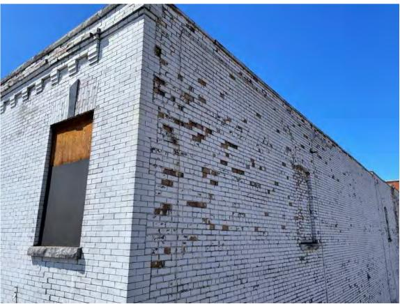
Photo 31: Exterior southeast corner – note the spalling brick due to moisture intrusion, freeze thaw cycles causes a spall, which falls to the ground.
