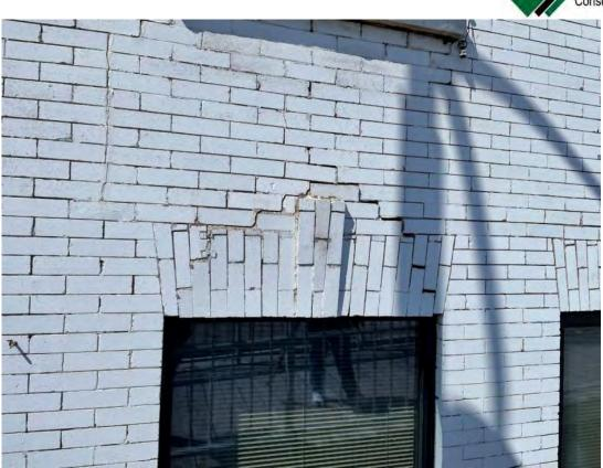
Photo 29: Typical exterior lintels are loose and failing and require replacement
