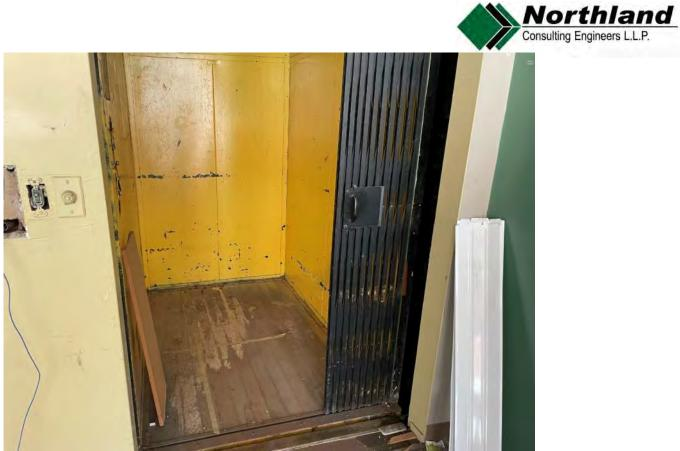
Photo 25: Existing freight elevator, would require significant upgrades or replacement if a significant renovation were to occur.
