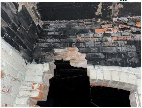
Photo 15: Existing sidewalk vault support is generally in poor condition
