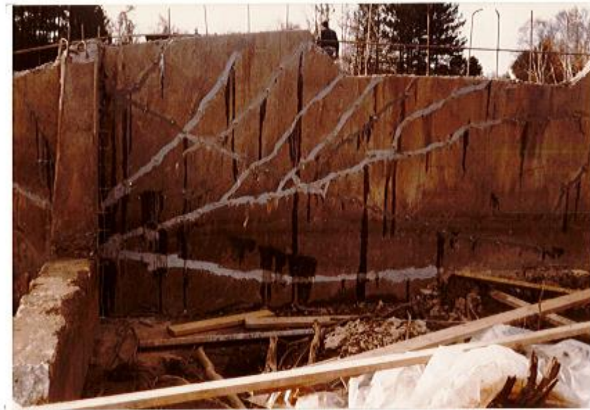
#11 10/16/85 FACE OF SOUTH WALL AFTER INJECTION
