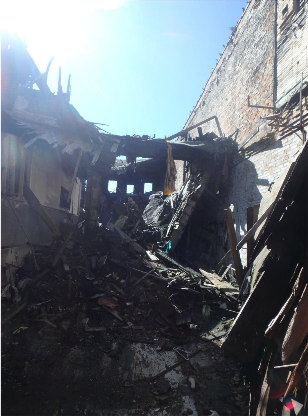
*View of the caved in roof of the 118 East 1<sup>st</sup> Street building which resulted from fire damage to the building sustained around Thanksgiving 2020.*
