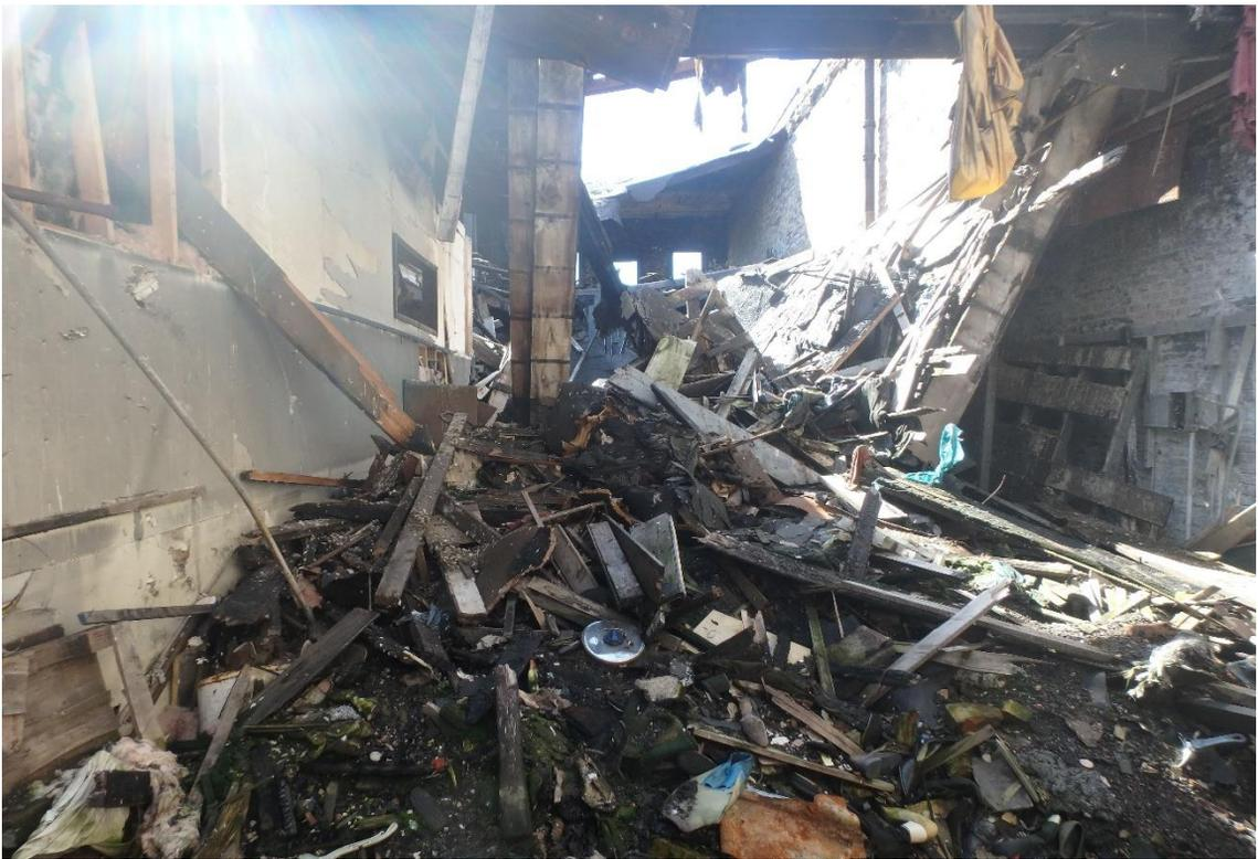
*Complete roof collapse and partial collapse of the second-floor structure of the 118 East 1<sup>st</sup> Street building.*
