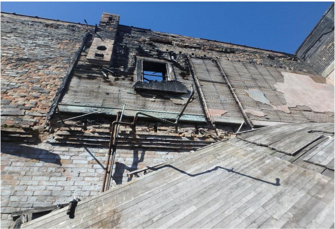
*Remaining interior wall feature (southwest side) of the 118 East 1<sup>st</sup> Street building showing fire and structural damage. Note roof absence and second floor separation.*
