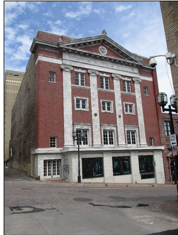
Photograph 5: View of the Classical Revival Orpheum Theatre on N. 2 nd Ave. E. Note the pediment, ionic pilasters, and keystone window lintels at the 3 d story.
