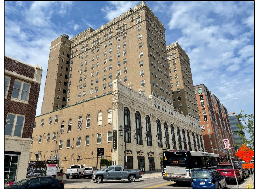
Photograph 9: View of the Italian Renaissance Revival Greysolon Plaza (Hotel Duluth) at the corner of E. Superior St. and N. 3rd Ave. E.
