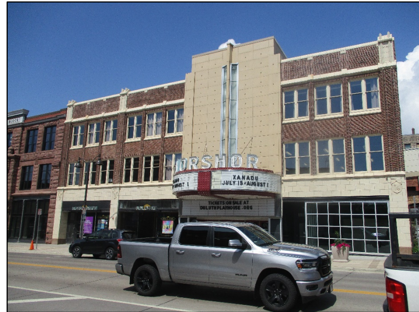
Photograph 8: View of the NorShor Theater with its Art Moderne marquee from a 1941 renovation.
