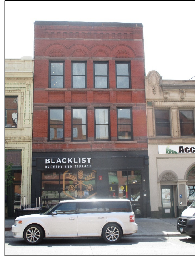
Photograph 7: View of the Italianate building at 120 E. Superior St.
