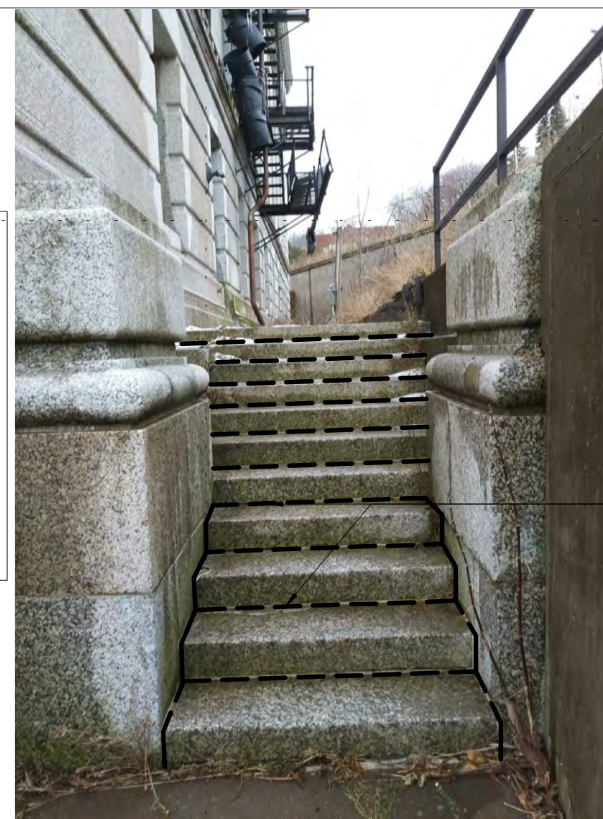
6 EXTERIOR STAIR AT NE CORNER
