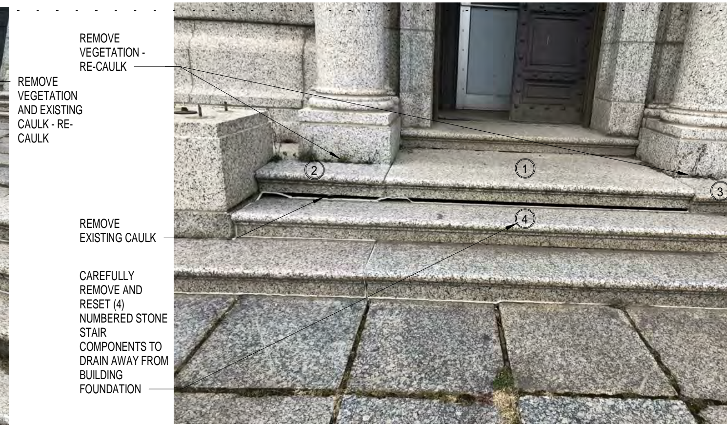
9 ENTRY STAIR - UPPER
