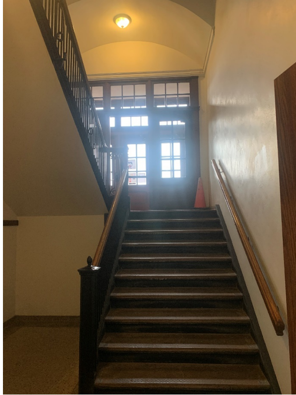
B.9 – Basement Photo 9: View from E looking W in West Stairway
