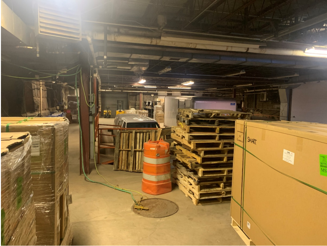
E.5 - Exterior Photo 5: View from E looking W in loading dock area
