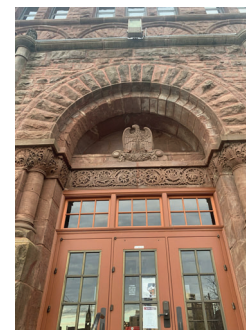
EFFLORESCENCE AND SPALLING AT ARCH, DEFLECTING STONES AND FAILED MORTAR JOINTS AT WASH PANEL ABOVE, SE ENTRANCE
