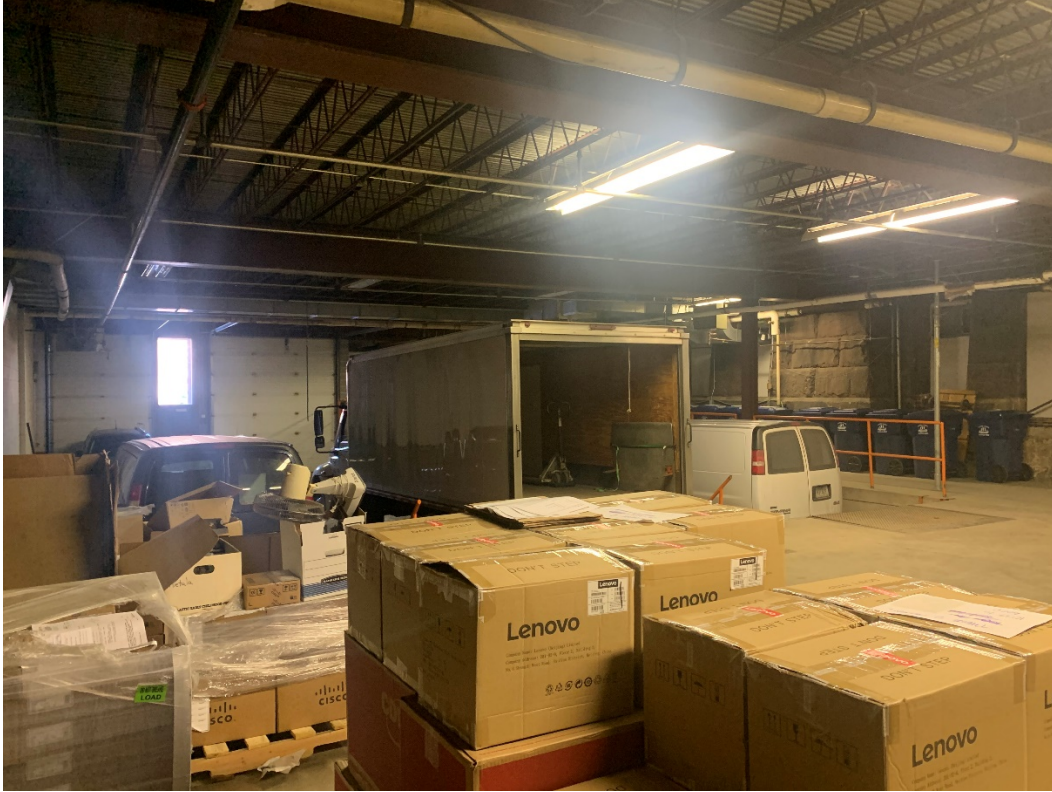
E.3 - Exterior Photo 3: View from NW looking SE in loading dock area
