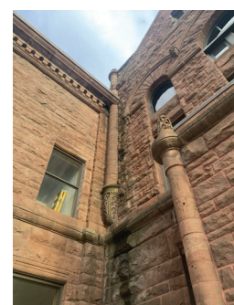
ADVANCED DETERIORATION AT THE HISTORIC DOWNSPOUT LOCATIONS
