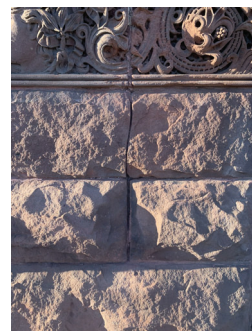
FAILED MORTAR JOINT AND CRACK
