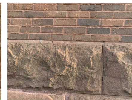
RUNNING CRACK AND FAILED MORTAR JOINTS AT BOILER HOUSE
