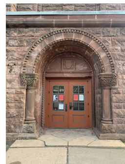
DIFFERENTIAL SETTLEMENT OF STONE LANDING AND ARCH EFFLORESCENCE AT MAIN N. ENTRANCE TO GYM
