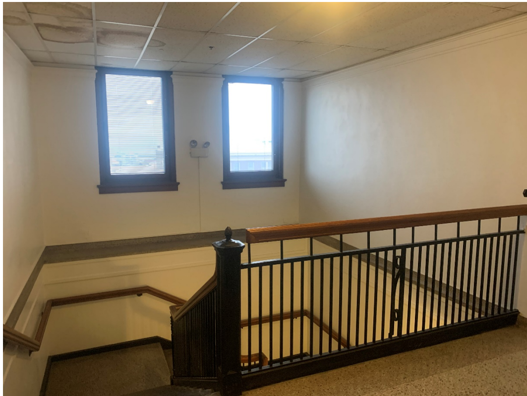
2.14 – Level Two Photo 14 – View from N looking S in South Stairway – West
