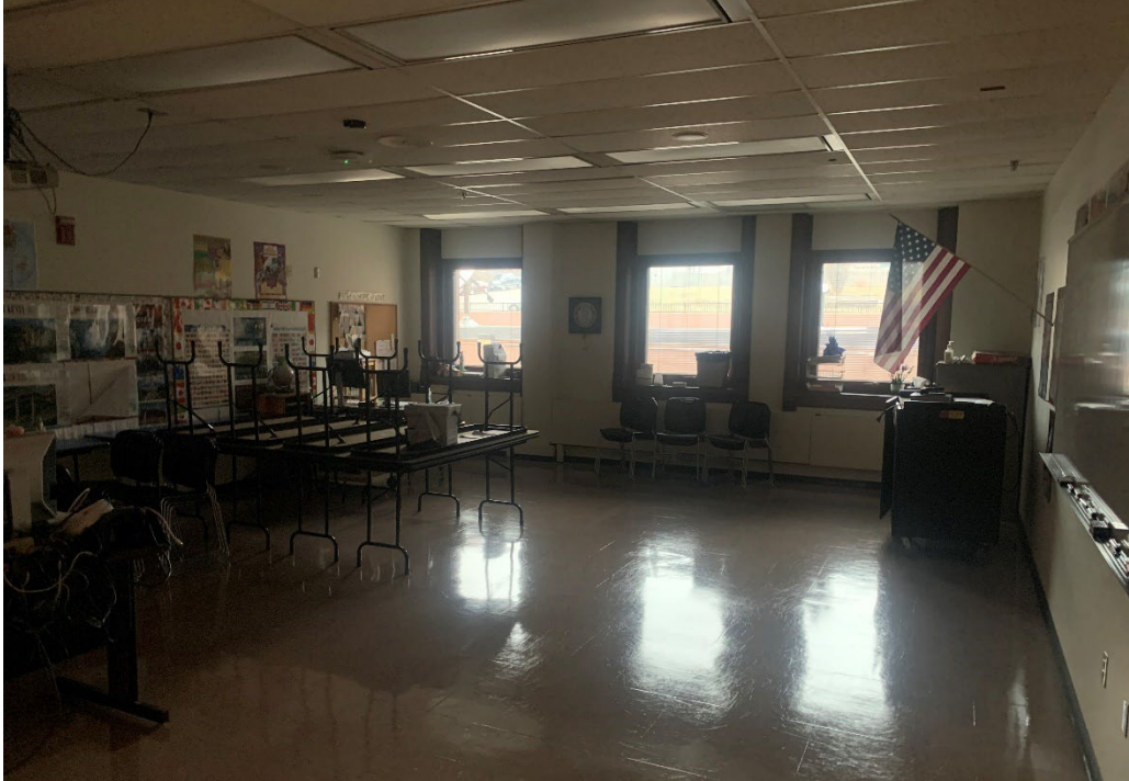
1.11 – Level One Photo 11 – View from SE looking NW into classroom
