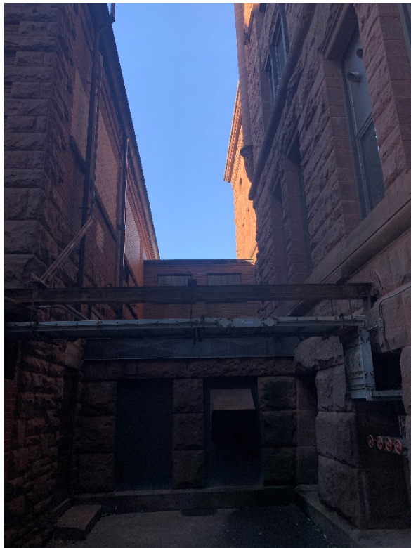
E.28 - Exterior Photo 28: View from S looking N at building connection
