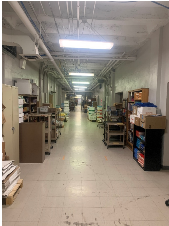
B.8 – Basement Photo 8: View from W looking E in corridor
