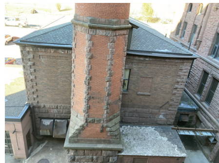
BOILER CHIMNEY - DETERIORATED MORTAR JOINTS ESPECIALLY ON THE HORIZONTAL SURFACES OF THE WASH PANEL
