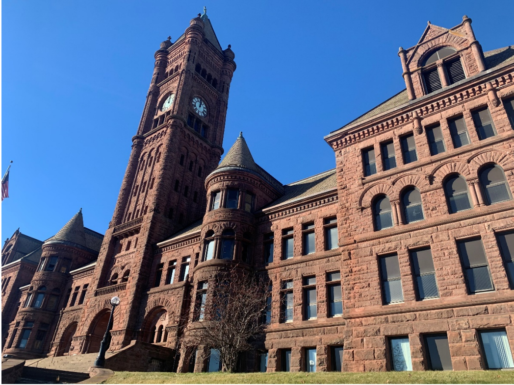
E.13 - Exterior Photo 13: View from SE looking NW at building
