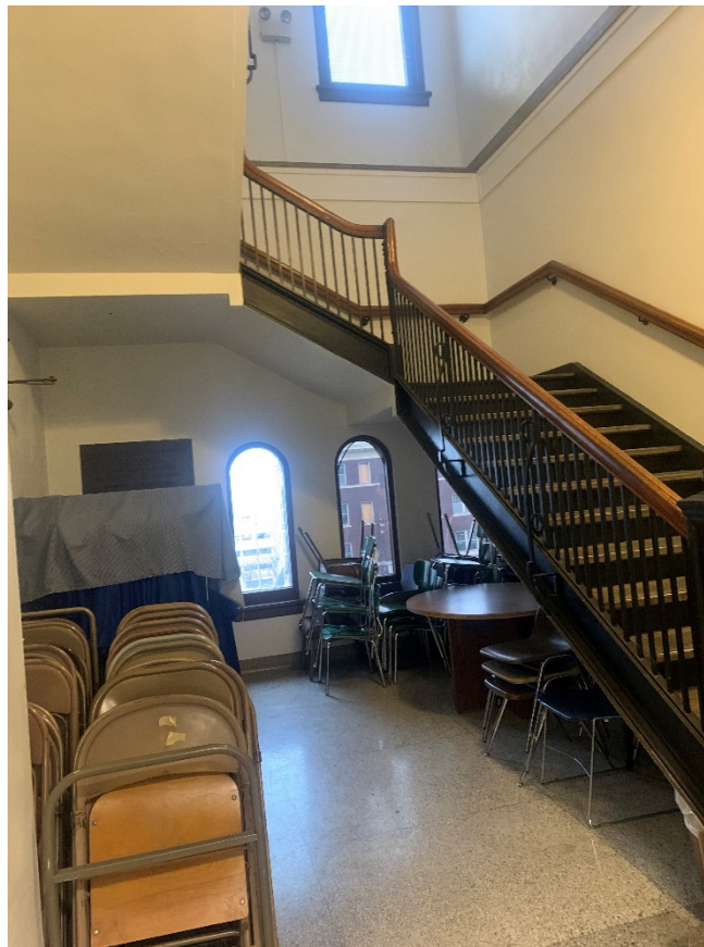
1.12 – Level One Photo 12 – View from N looking S into South Stairwell – West
