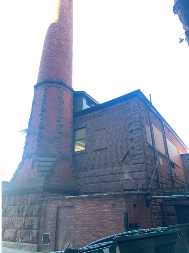
E.27 - Exterior Photo 27: View from SE looking NW at chimney
