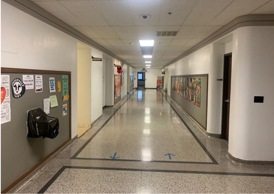
3.7 – Level Three Photo 7 – View from E looking W in E/W Corridor
