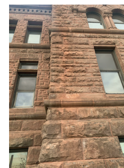
ADVANCED DETERIORATION AT THE HISTORIC DOWNSPOUT LOCATIONS
