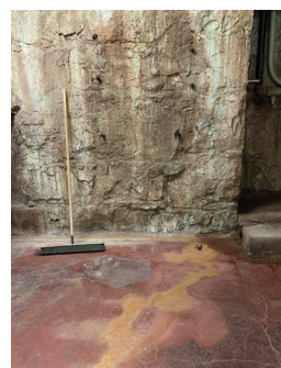
FOUNDATION WALL IN BOILER ROOM
