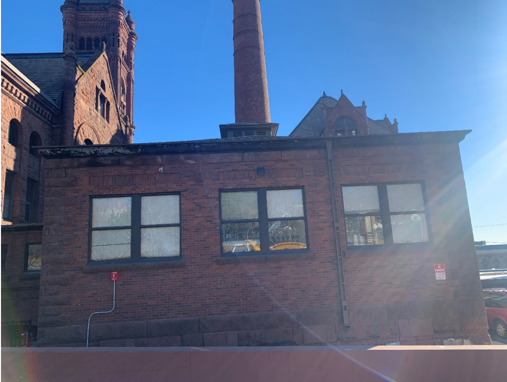
E.31 - Exterior Photo 31: View from N looking S at building
