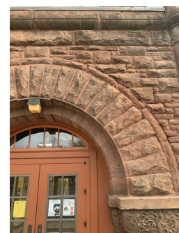
BADLY DETERIORATED MORTAR JOINTS AND DEFLECTING STONES AT TOP OF ARCH, MAIN N. ENTRANCE
