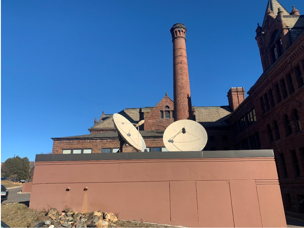
E.29 - Exterior Photo 29: View from W looking E at garage and building
