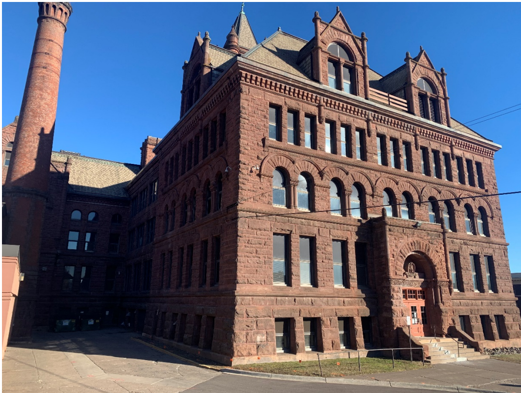
E.22 - Exterior Photo 22: View from NW looking SE at West Entrance
