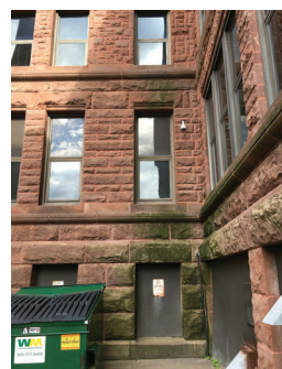
IDENTIFY GENERAL NATURE AND SOURCE OF HEAVY SOILING IN WEST DOCK.
