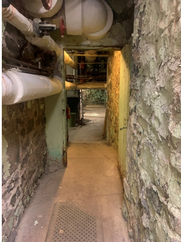
B.17 – Basement Photo 17: View from E looking W in machine room hallway
