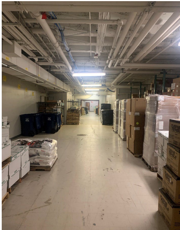
B.4 – Basement Photo 4: View from W looking E in corridor
