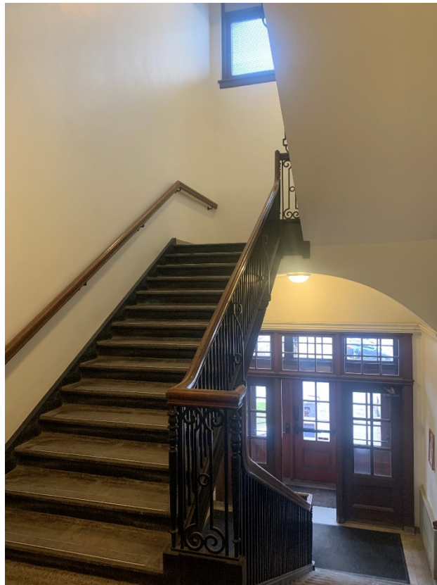
1.2 – Level One Photo 2 – View from W looking E into east stairway
