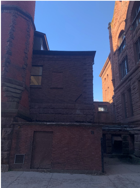
E.26 - Exterior Photo 26: View from S looking N at building connection
