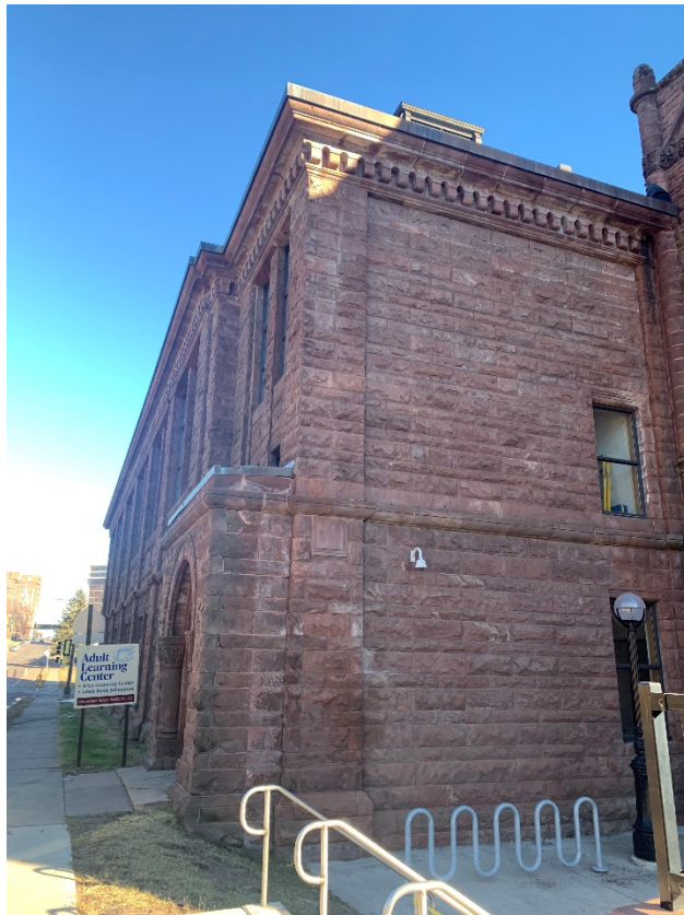
E.34 - Exterior Photo 34: View from NW looking SE at Gym Addition
