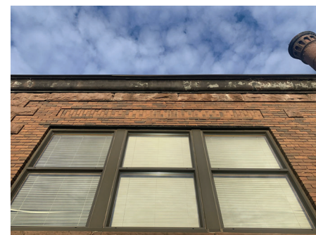
EFFLORESCENCE AT CORNICE LIKELY DUE TO ROOF LEAKAGE AND TYPICAL BRICK FACADE
