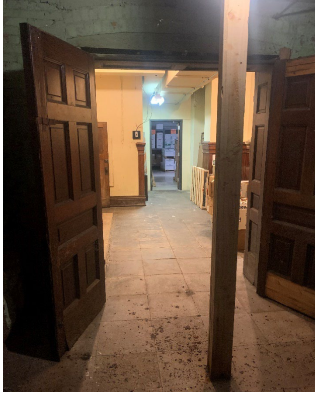
B.13 – Basement Photo 13: View from S looking N from storage room
