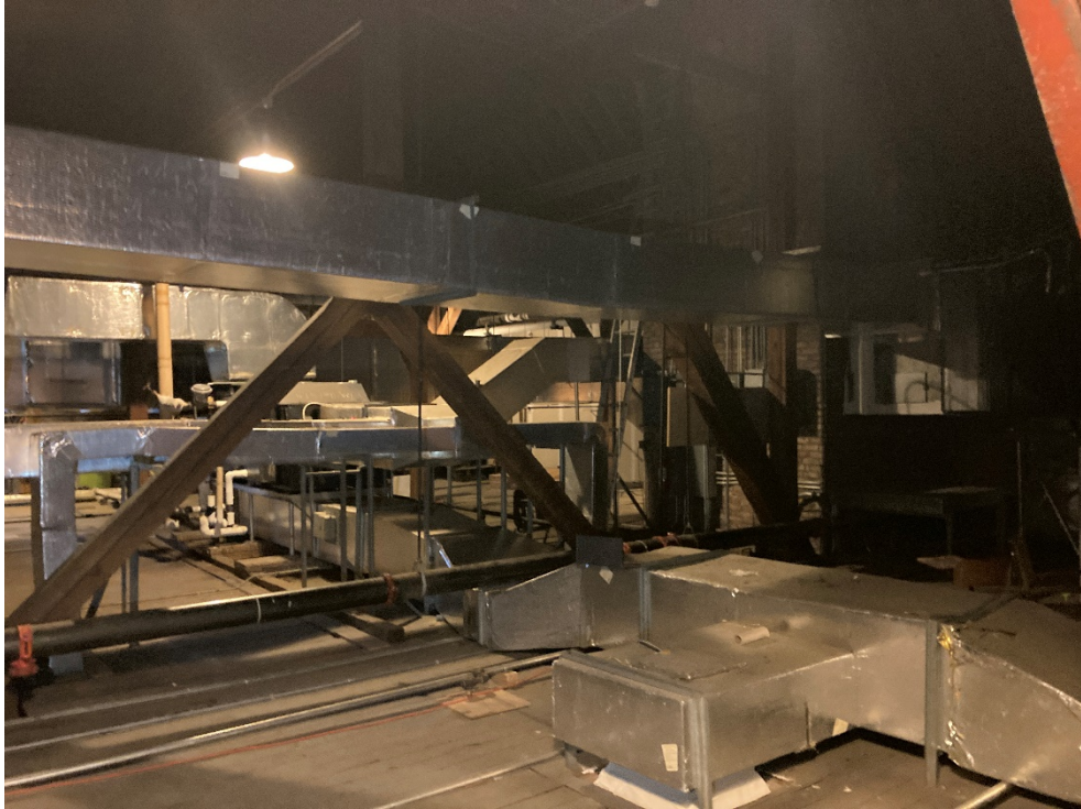
4.1 – Level Four Photo 1 – View from NE looking SW in attic
