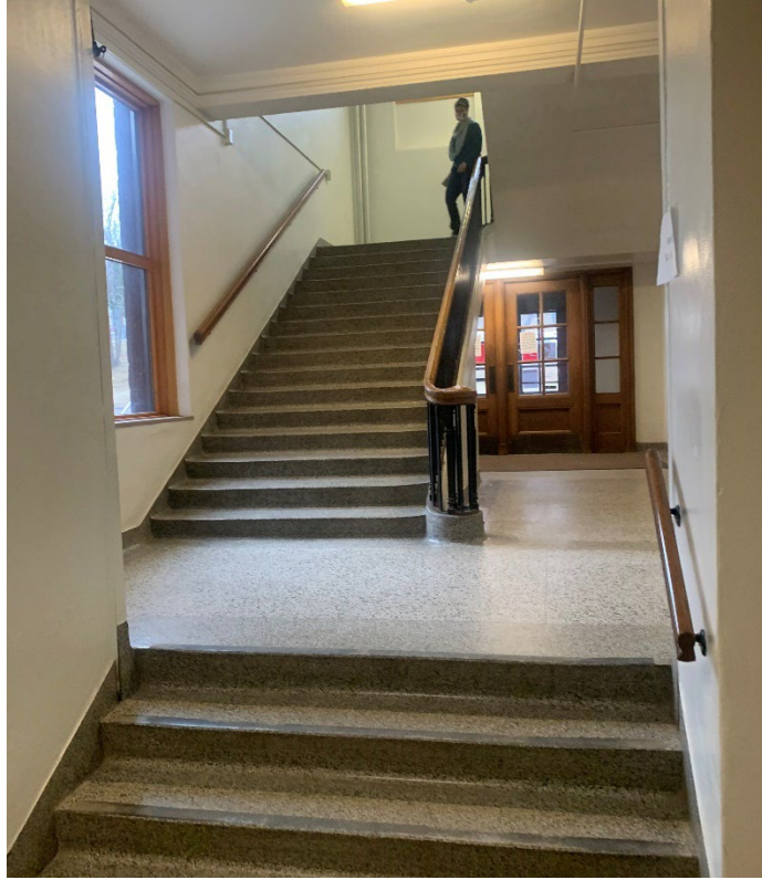
1.19 – Level One Photo 19 – View from S looking N at North Stairs
