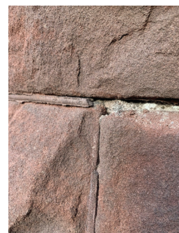
TYPICAL FAILED MORTAR JOINT
