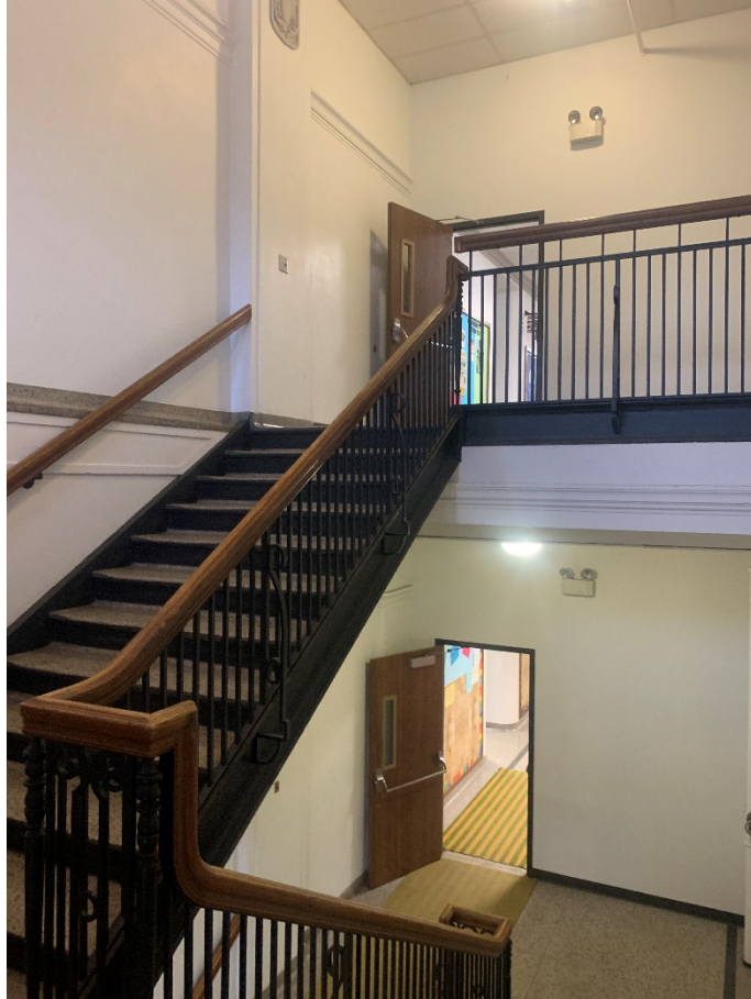
2.21 – Level Two Photo 21 – View from E looking W in East Stairway
