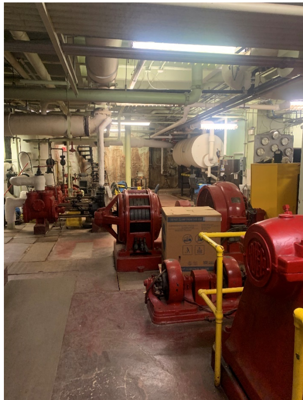
B.16 – Basement Photo 16: View from S looking N in machine room
