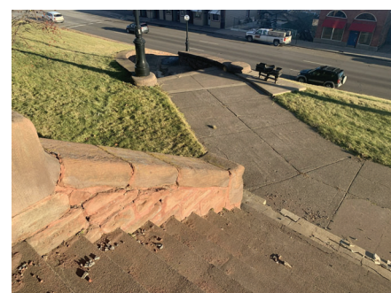
BALUSTRADE AND CONC. STAIRS IN POOR CONDITION, SIMILAR BEYOND AT CURVED STAIR AND BALUSTRADE.
