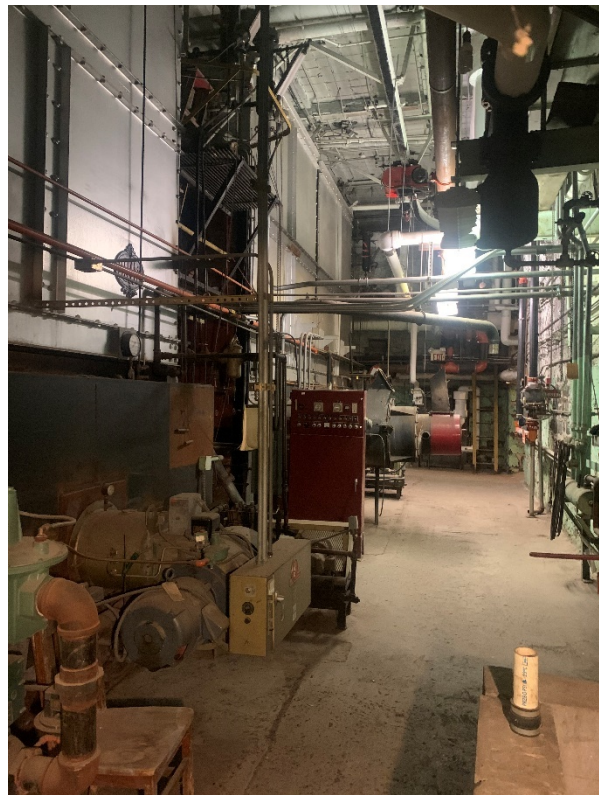
B.18 – Basement Photo 18: View from SE looking NW in machine room
