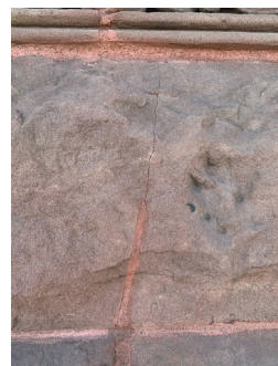
CRACKING. NOTE INAPPROPRIATE PINK MORTAR FOUND THROUGHOUT
