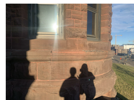
IMPROPER MORTAR PATCHING ON WASH PANEL
