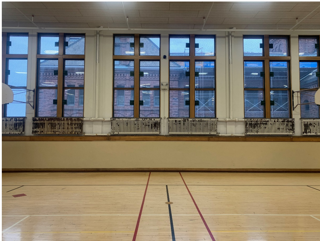
2.4 – Level Two Photo 4 – View from N looking S in Gym
