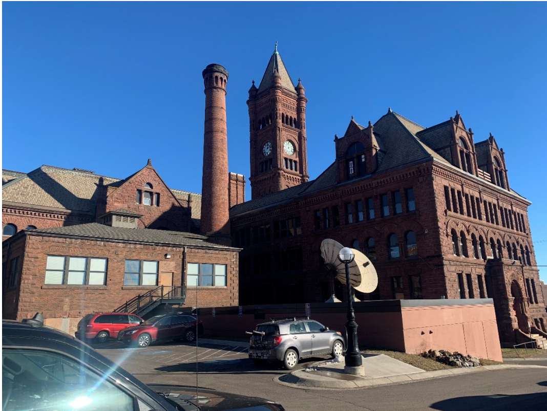
E.30 - Exterior Photo 30: View from NW looking SE at building
