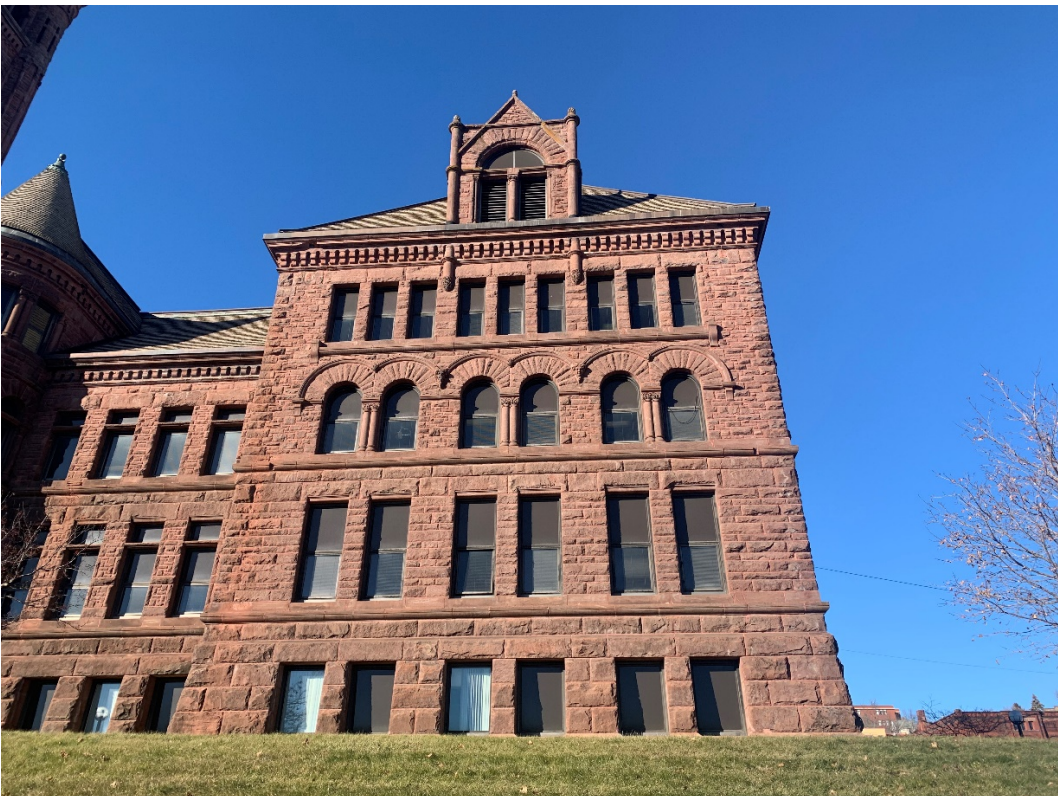
E.12 - Exterior Photo 12: View from S looking N at building
