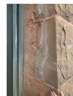
TYPICAL EFFLORESCENCE AND SPALLING AT MASONRY OPENINGS
