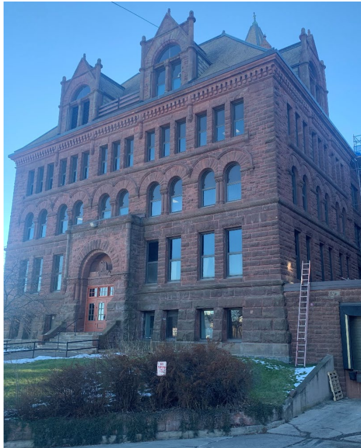
E.8 - Exterior Photo 8: View from NE looking SW at East Entrance
