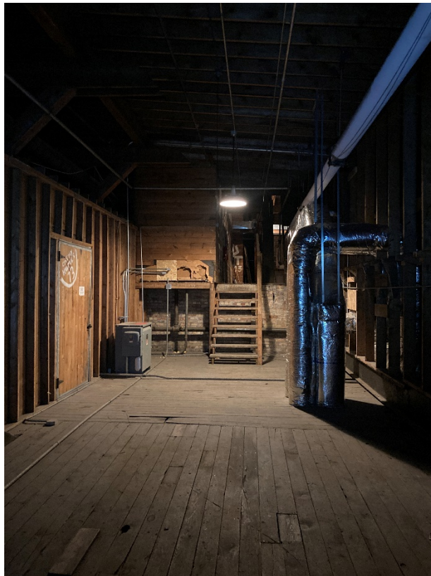
4.2 – Level Four Photo 2 – View from E looking W in attic
