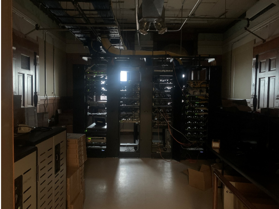
2.15 – Level Two Photo 15 – View from N looking S in room within Belltower
