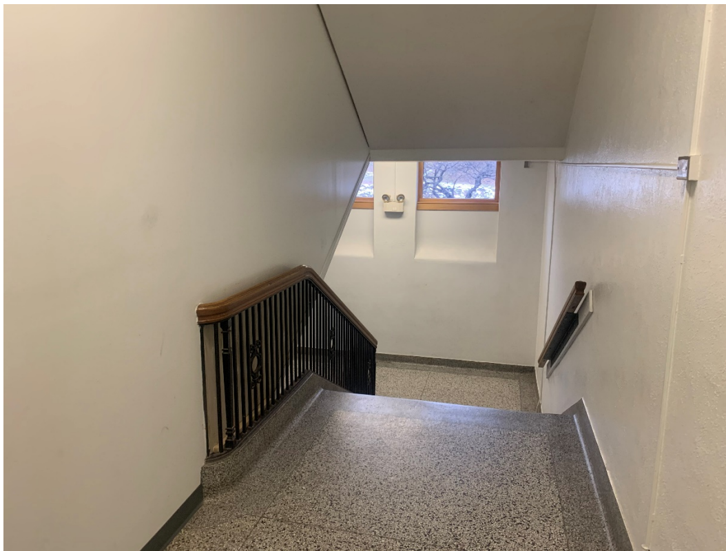
2.6 – Level Two Photo 6 – View from S looking N down North Stairs
