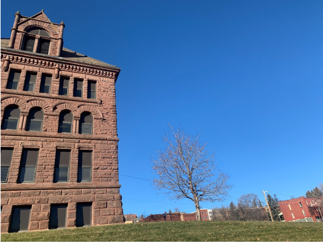
E.11 - Exterior Photo 11: View from S looking N at building
