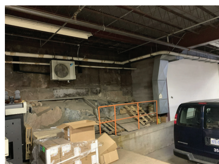
FOUNDATION WALL UNDER GYMNASIUM ON BEDROCK IN EAST DOCK
