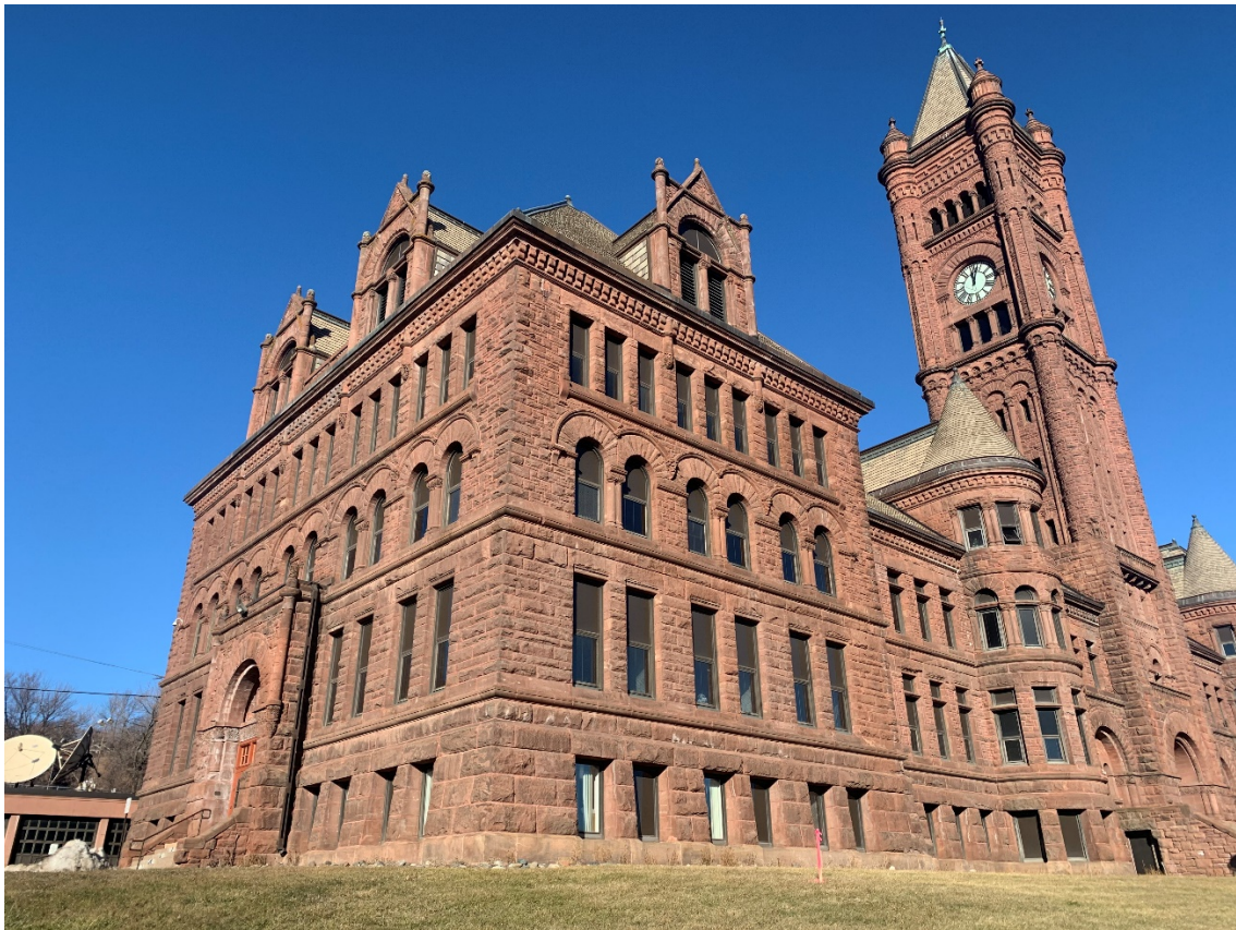
E.20 - Exterior Photo 20: View from SW looking NE at building
