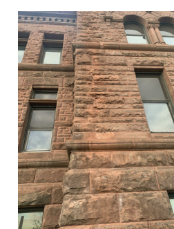
ADVANCED DETERIORATION AT THE HISTORIC DOWNSPOUT LOCATIONS
