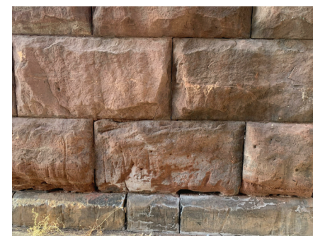
BASE OF CHIMNEY, EVIDENCE OF WATER INFILTRATION, FAILED MORTAR JOINTS, AND DAMAGED STONE.
