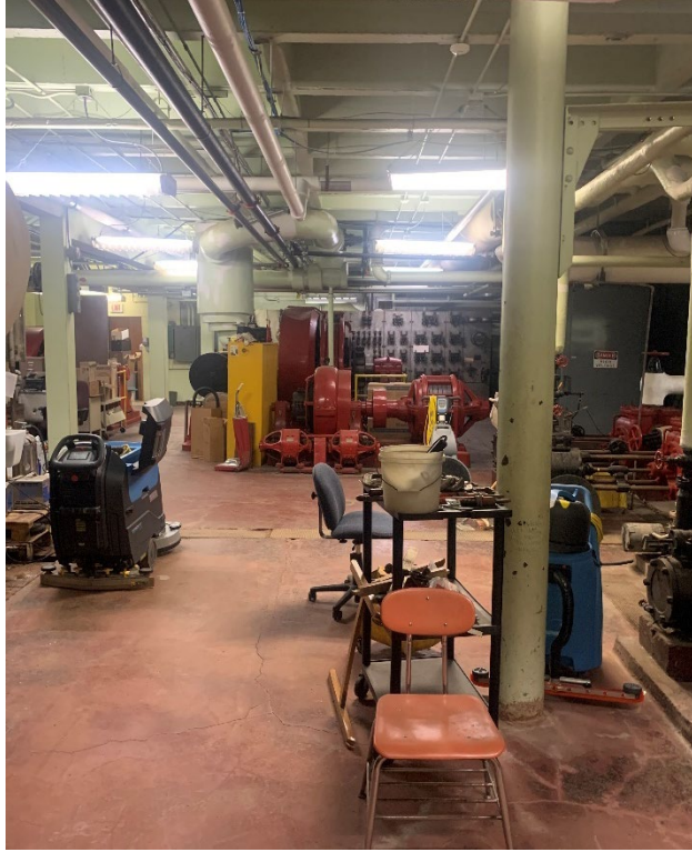
B.15 – Basement Photo 15: View from N looking S into machine room
