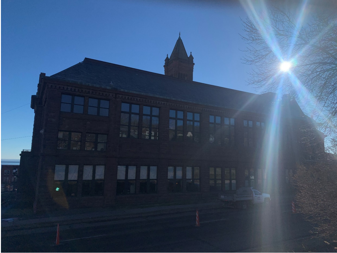
E.35 - Exterior Photo 35: View from N looking S at Gym Addition
