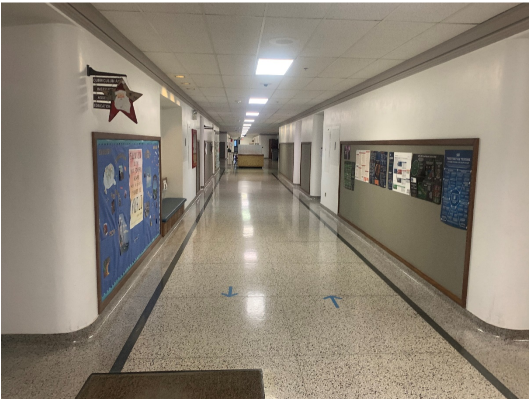
3.2 – Level Three Photo 2 – View from E looking W in E/W Corridor
