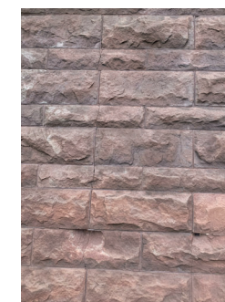
TYPICAL RUNNING CRACK
