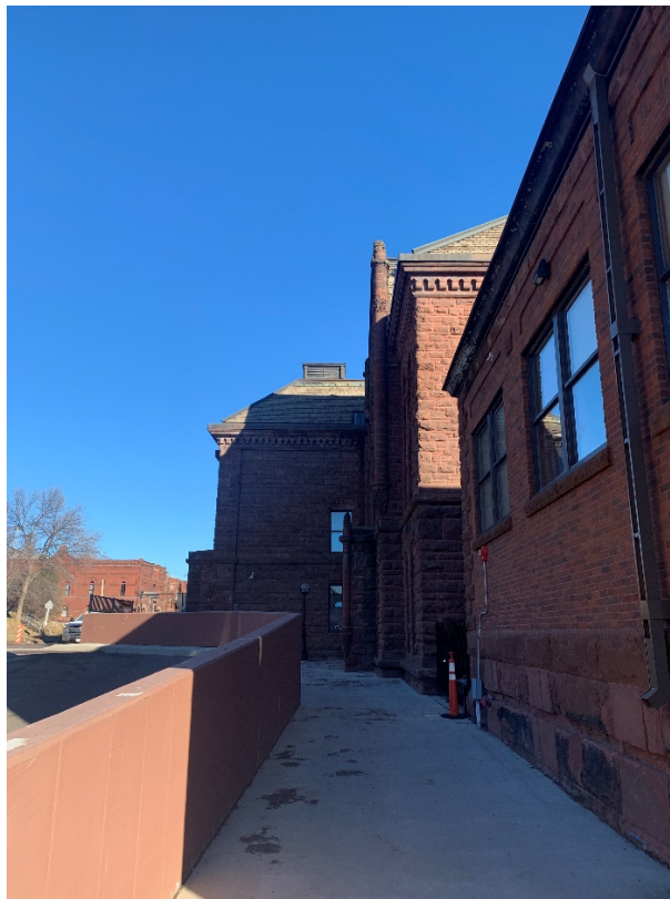
E.32 - Exterior Photo 32: View from E looking W at building from sidewalk
