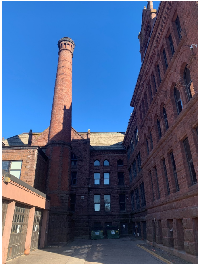
E.24 - Exterior Photo 24: View from W looking E at alley area
