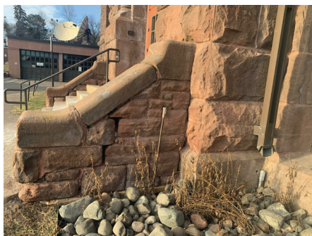
BALUSTRADE IN POOR CONDITION
