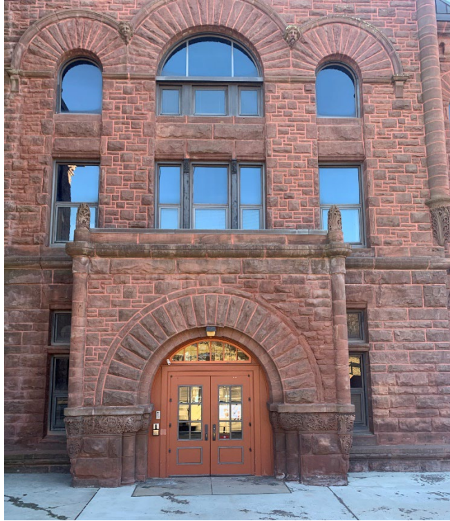
E.33 - Exterior Photo 33: View from N looking S at North Entrance
