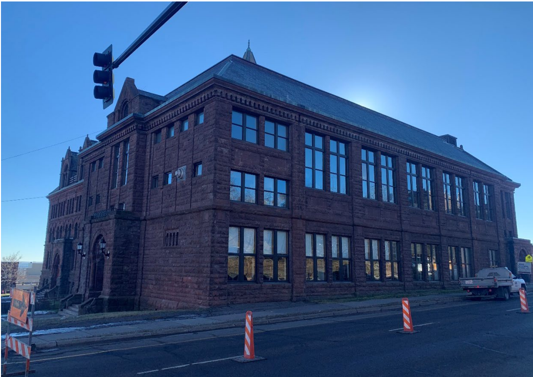
E.36 - Exterior Photo 36: View from NE looking SW at Gym Addition
