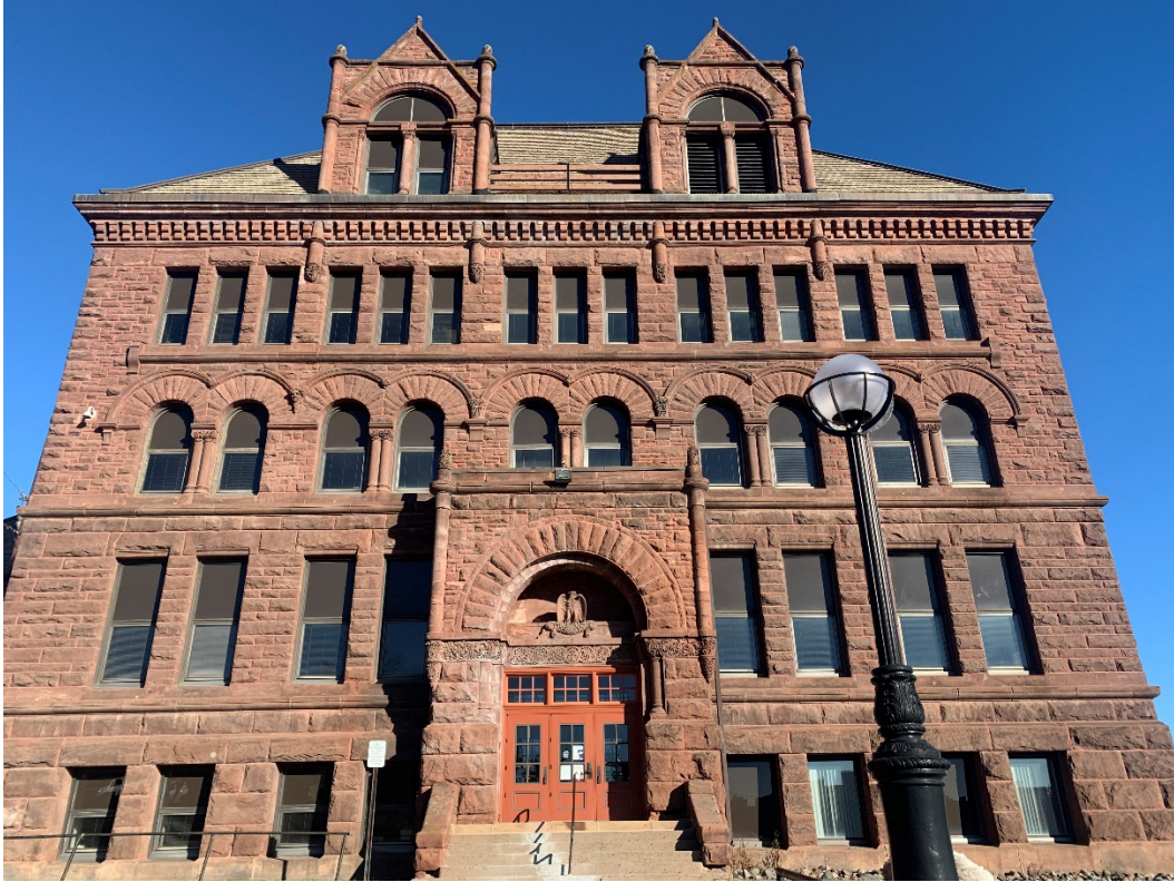
E.21 - Exterior Photo 21: View from W looking E at West Entrance
