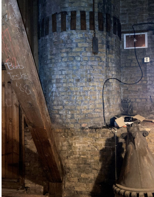
4.3 - Level Four Photo 3 – View from N looking S in attic
