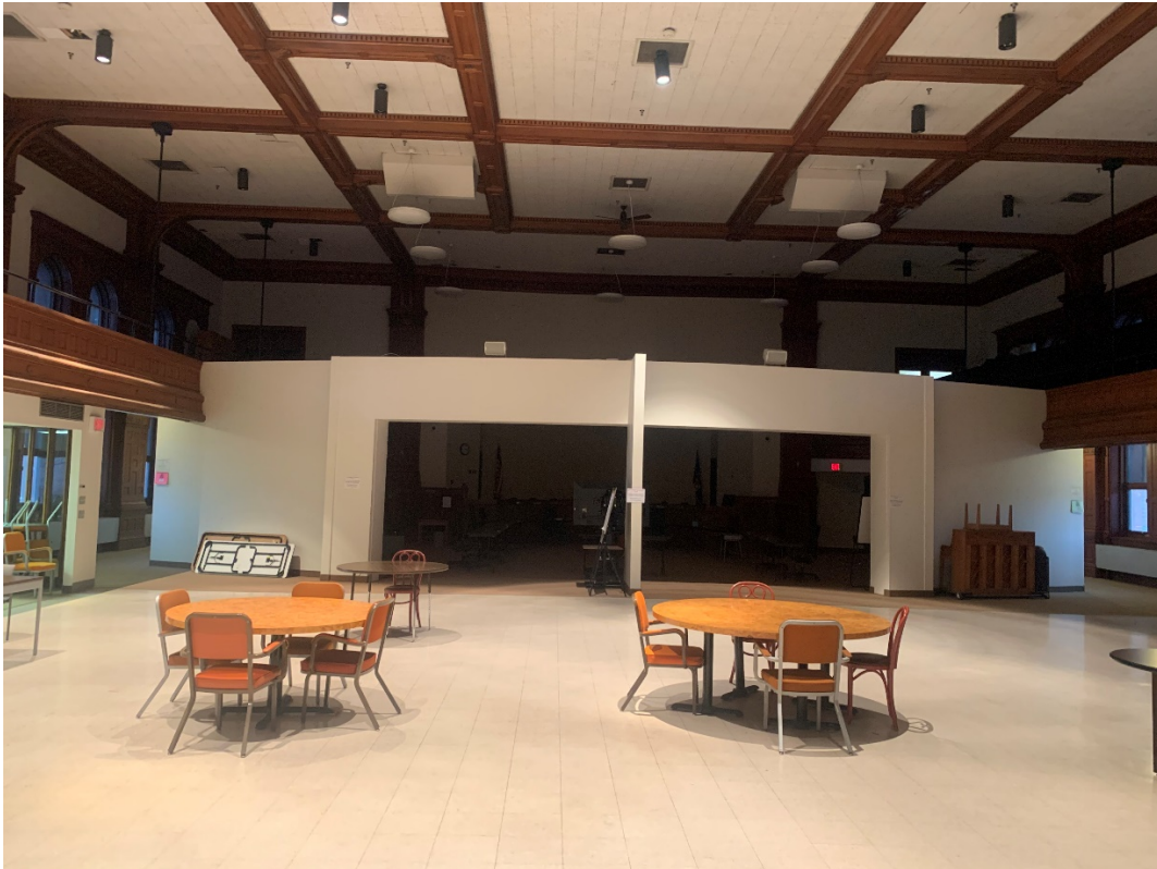
2.8 – Level Two Photo 8 – View from N looking S in Auditorium
