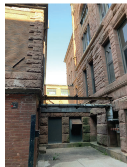
STEEL ANCHORS CAUSING CRACKING AND SPALLING IN WEST DOCK.
