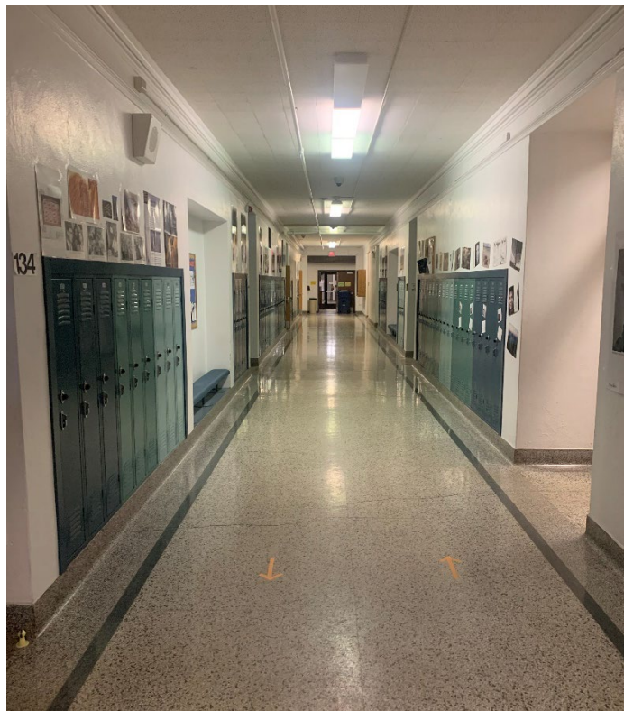
1.20 – Level One Photo 20 – View from E looking W down corridor at Gym Addition
