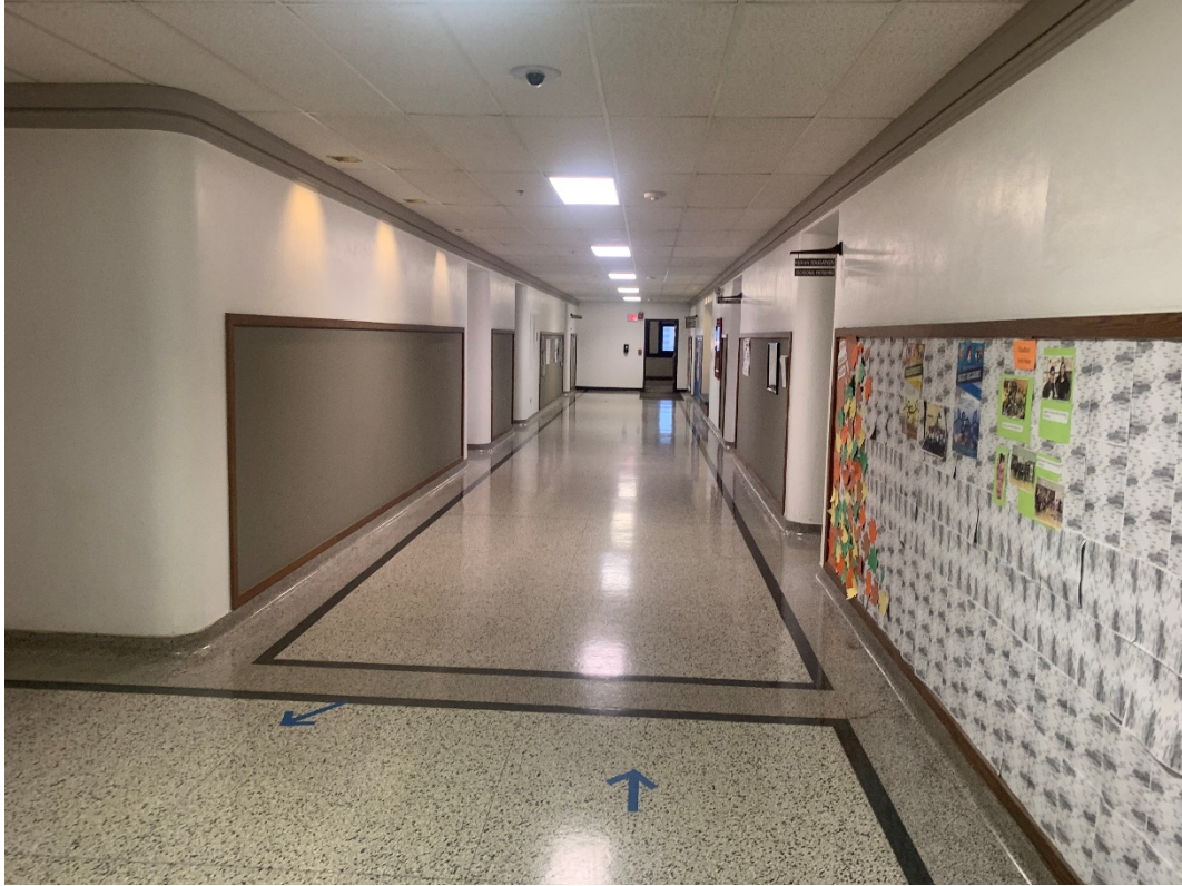
3.5 – Level Three Photo 5 – View from W looking E in E/W Corridor
