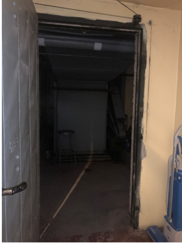
B.19 – Basement Photo 19: View from S looking N into storage room
