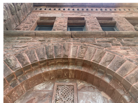
EFFLORESCENCE AND SPALLING AT ARCH. DEFLECTING STONES AND FAILED MORTAR JOINTS AT WASH PANEL ABOVE.
