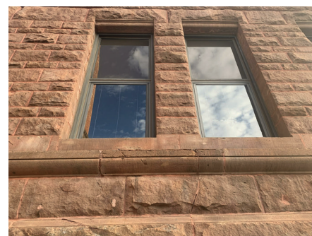
CRACKING AND SPALLING AT WASH LEDGE
