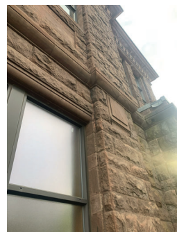
NOTE EFFLORESCENCE AT THE UPPER SOFFIT
