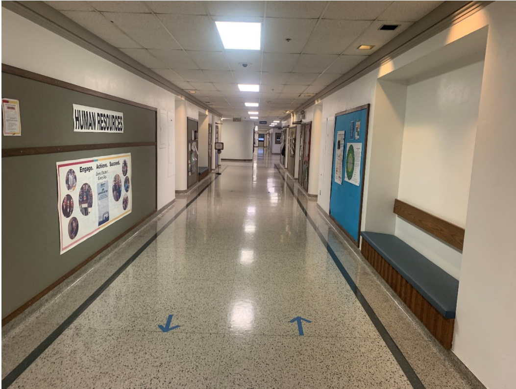
2.17 – Level Two Photo 17 – View from W looking E in E/W Corridor
