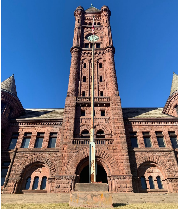
E.15 - Exterior Photo 15: View from S looking at clock tower
