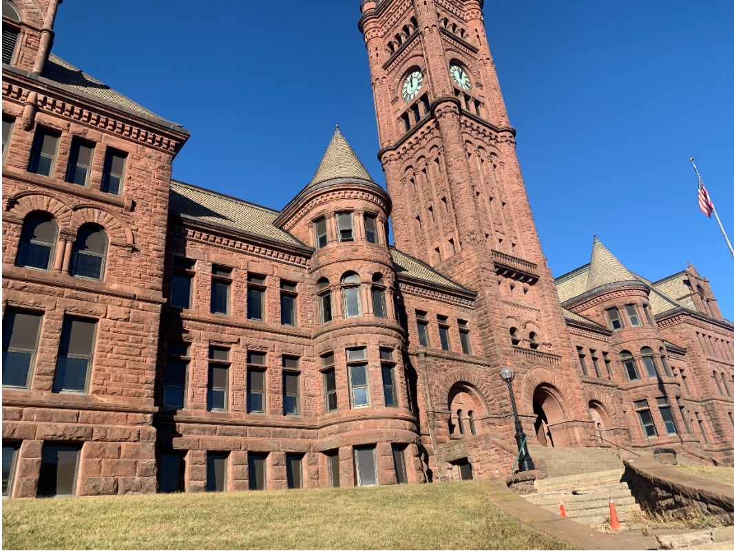
E.17 - Exterior Photo 17: View from SW looking NE at building
