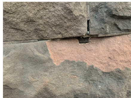
DETERIORATING STEEL CAUSING DAMAGE
