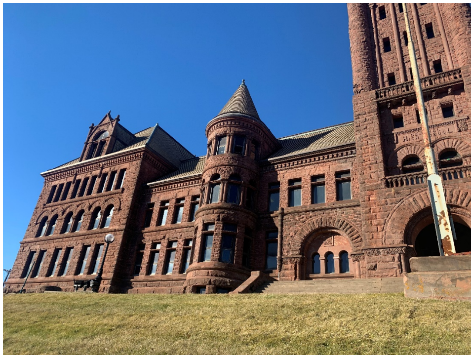
E.16 - Exterior Photo 16: View from SE looking NW at building
