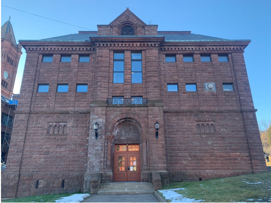
E.37 - Exterior Photo 37: View from E looking W at Gym Addition
