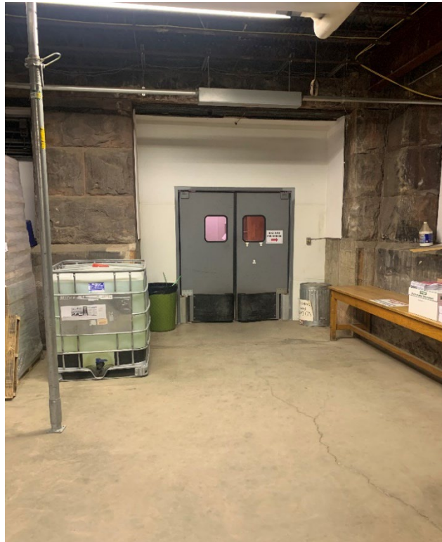
E.1 - Exterior Photo 1: View from N looking S in loading dock area
