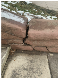
BALUSTRADE IN POOR CONDITION
