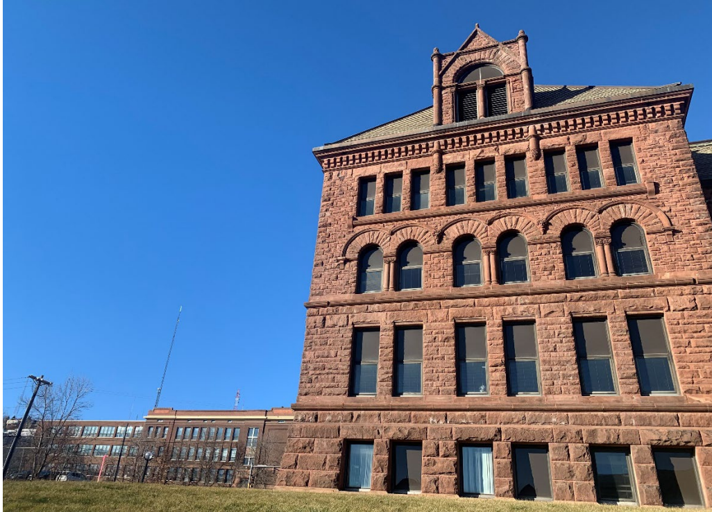
E.19 - Exterior Photo 19: View from S looking N at building
