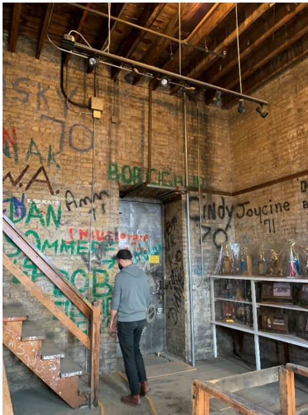
4.4 Clocktower at Attic Level, standing from SW looking NE
