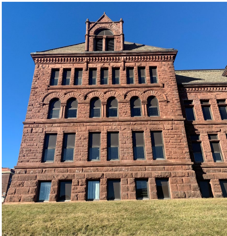
E.18 - Exterior Photo 18: View from S looking N at building
