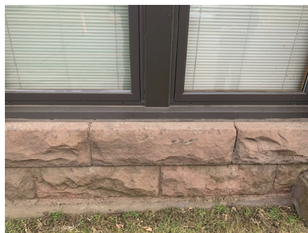
FAILED MORTAR JOINTS
