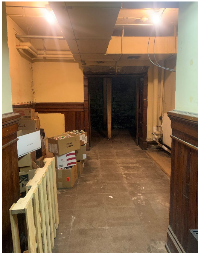
B.12 – Basement Photo 12: View from N looking S into storage room
