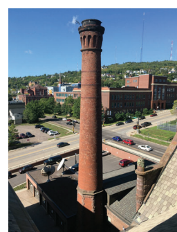
BOILER HOUSE CHIMNEY, NOTE RESILIENT TREE
