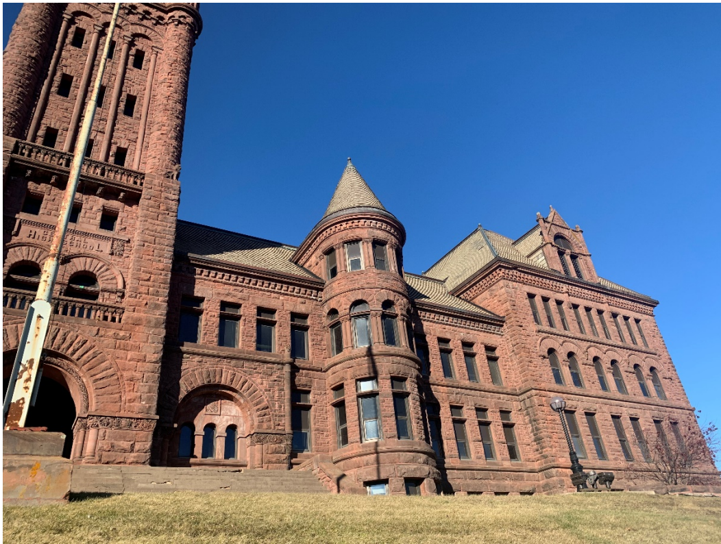
E.14 - Exterior Photo 14: View from SW looking NE at building
