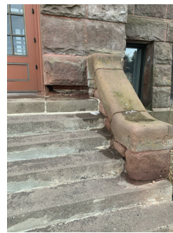
NOTE SEVERE DETERIORATION AT STONE BASE ON SE LANDING
