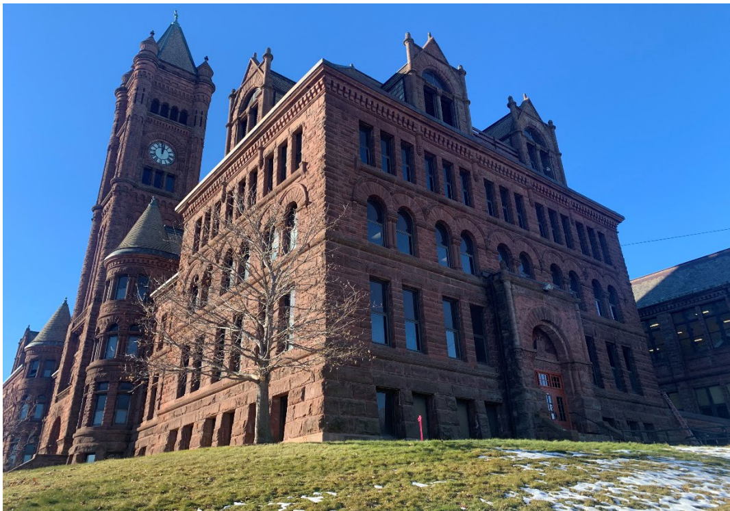
E.10 - Exterior Photo 10: View from SE looking NW at building
