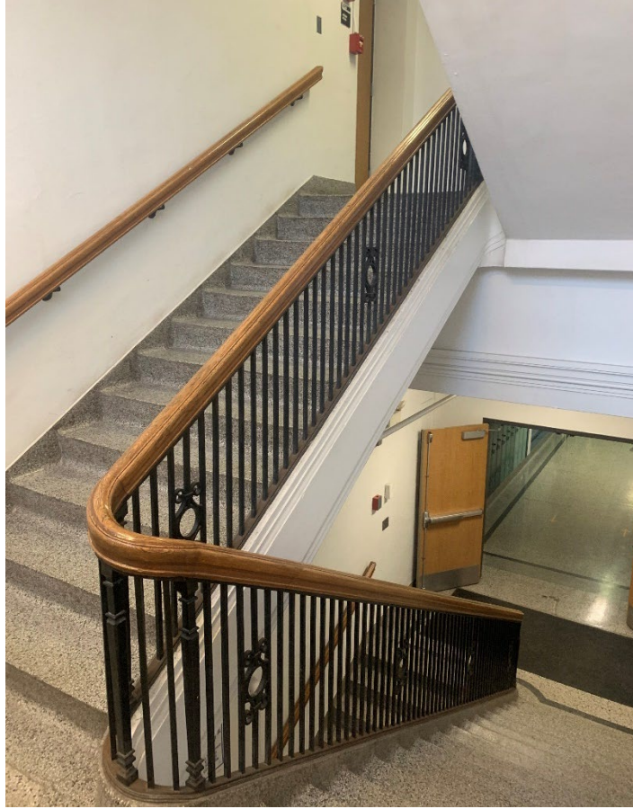
2.1 – Level Two Photo 1 – View from NE looking SW in East stairs at Gym
