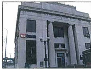
Corridor Building II
