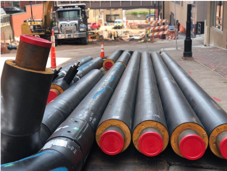
hot water pipes waiting to be installed
