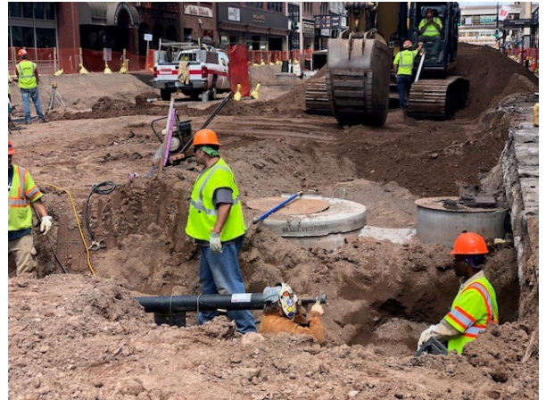
Crew installing hot water pipes
