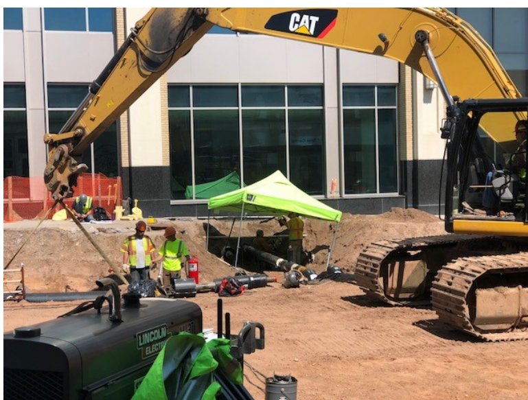
Crews installing hot water to maurices
