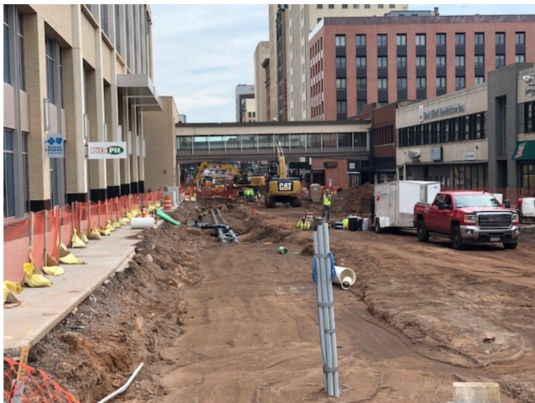
View from 5th Ave West (gray tubes are for electrical wires)
