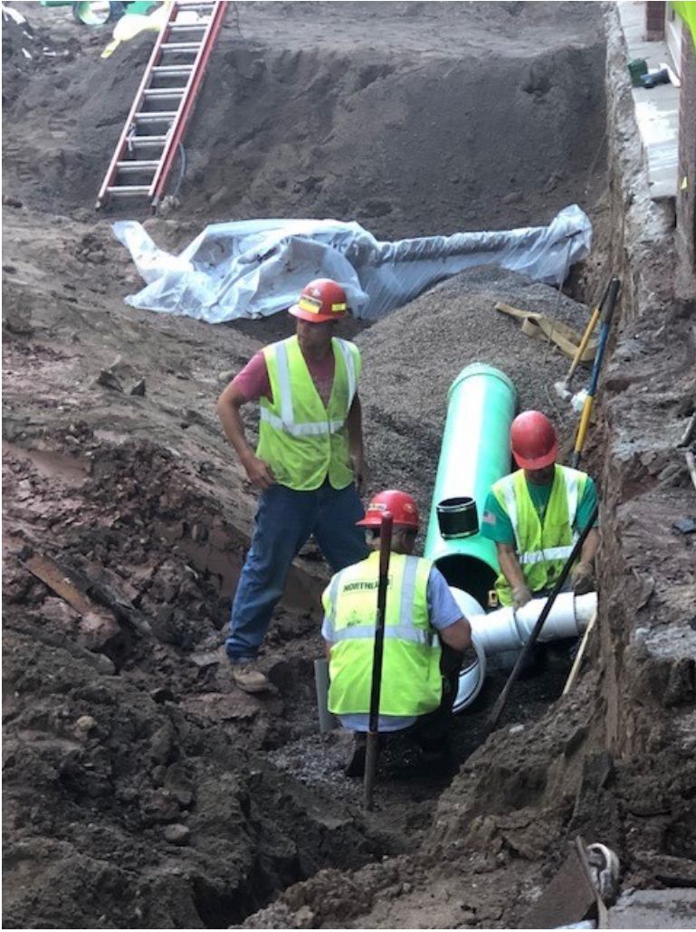
crews installing water line
