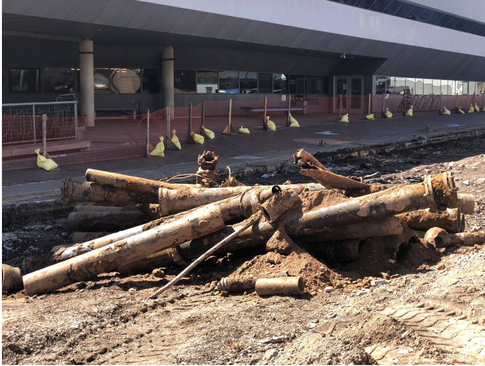
old water main excavated in front of Duluth Library
