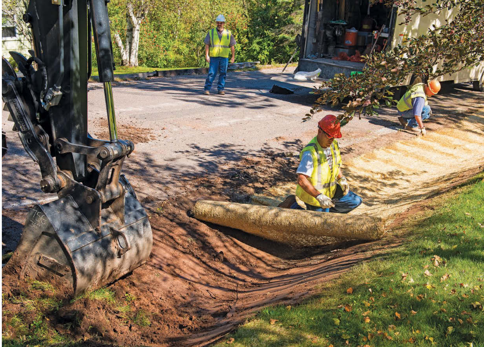
A crew from the Duluth Utility Operations Division recontours a ditch for stormwater conveyance.
