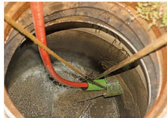
Clockwise from left: Erick Fronden removes a manhole lid to investigate a potential I&I issue as Todd Carlson looks on; Chris Anderson checks the controls of the Vactor 2100 while cleaning a sewer line with Erick Fronden and Brice Aikin ; a look down the manhole with the jetter hose inside the sewer line.
