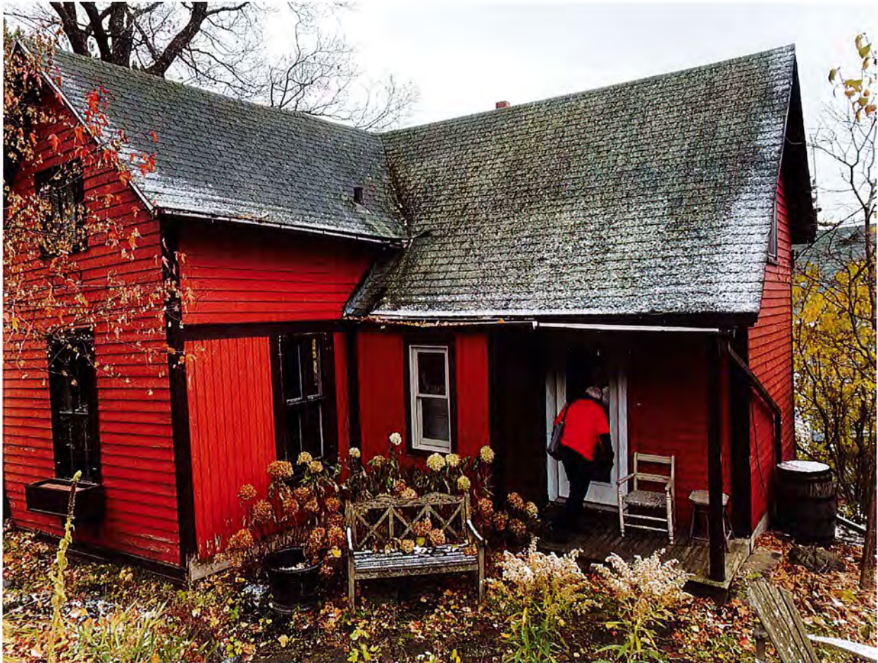
Image 4. North-Northwestern side of building
