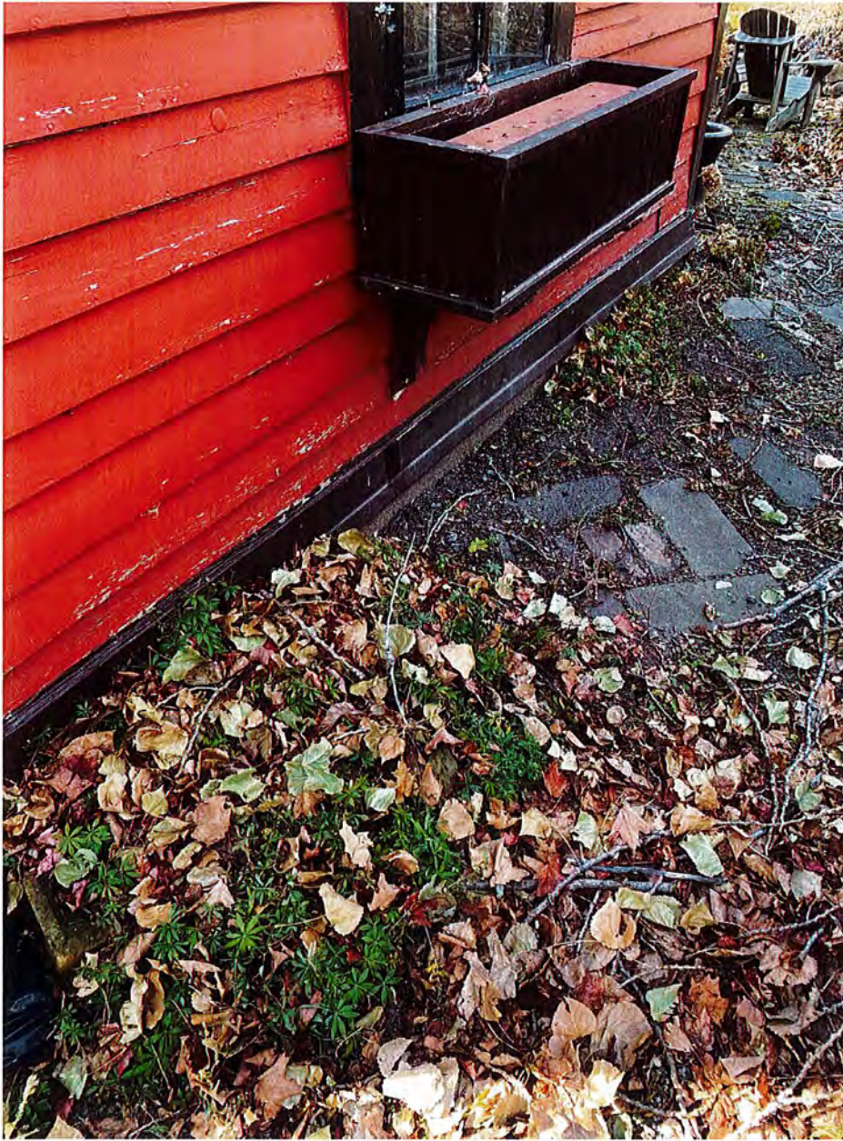
Image 2. Northern side of building
