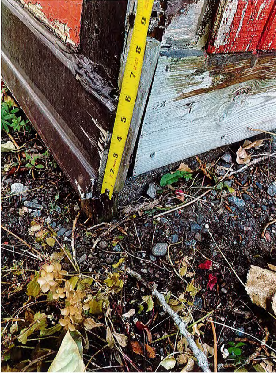
Image 3. NW corner of dining room; showing rim board/grade condition
