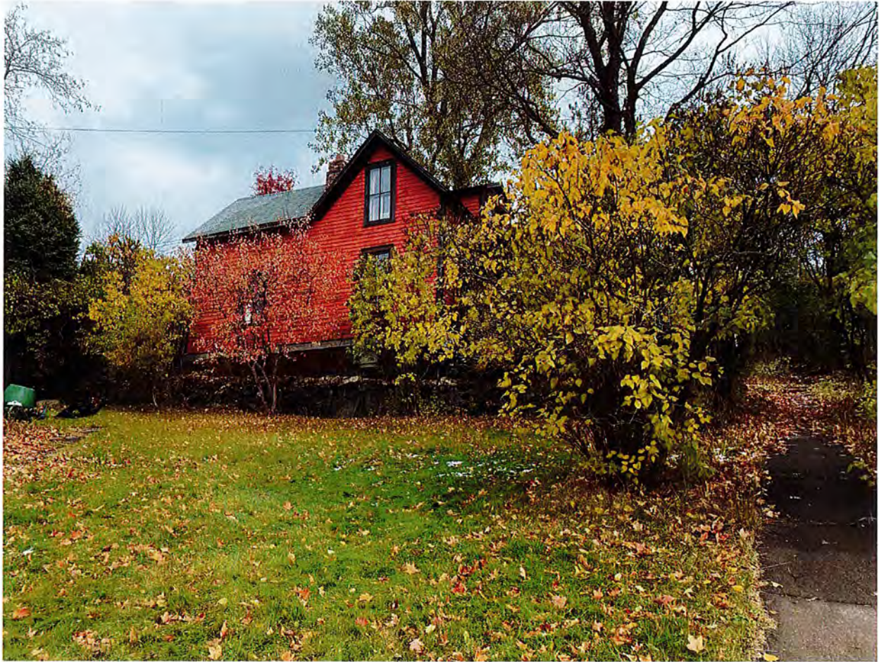
Image 5. Southern side of building
