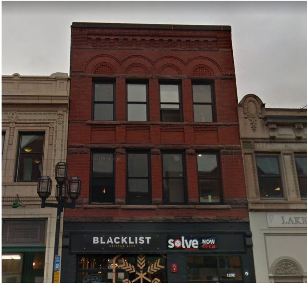
Street view of the upper floors
