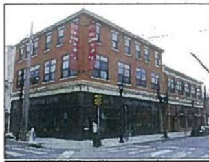
Main Street Building II
