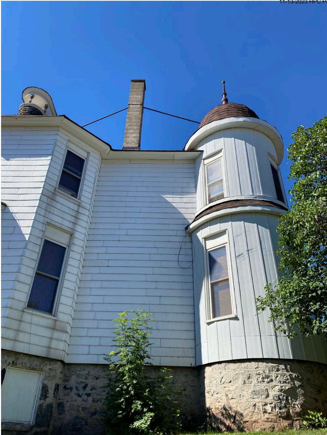
Photo 0015: View of tower, chimney, and dormer at the east elevation, looking west.
