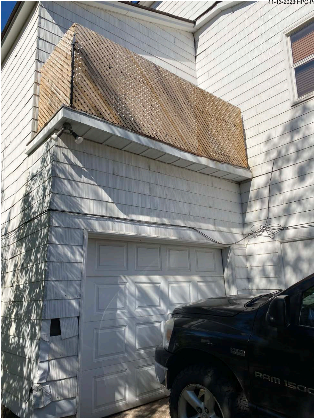
Photo 0014: View of garage entrance at east elevation, looking northwest.
