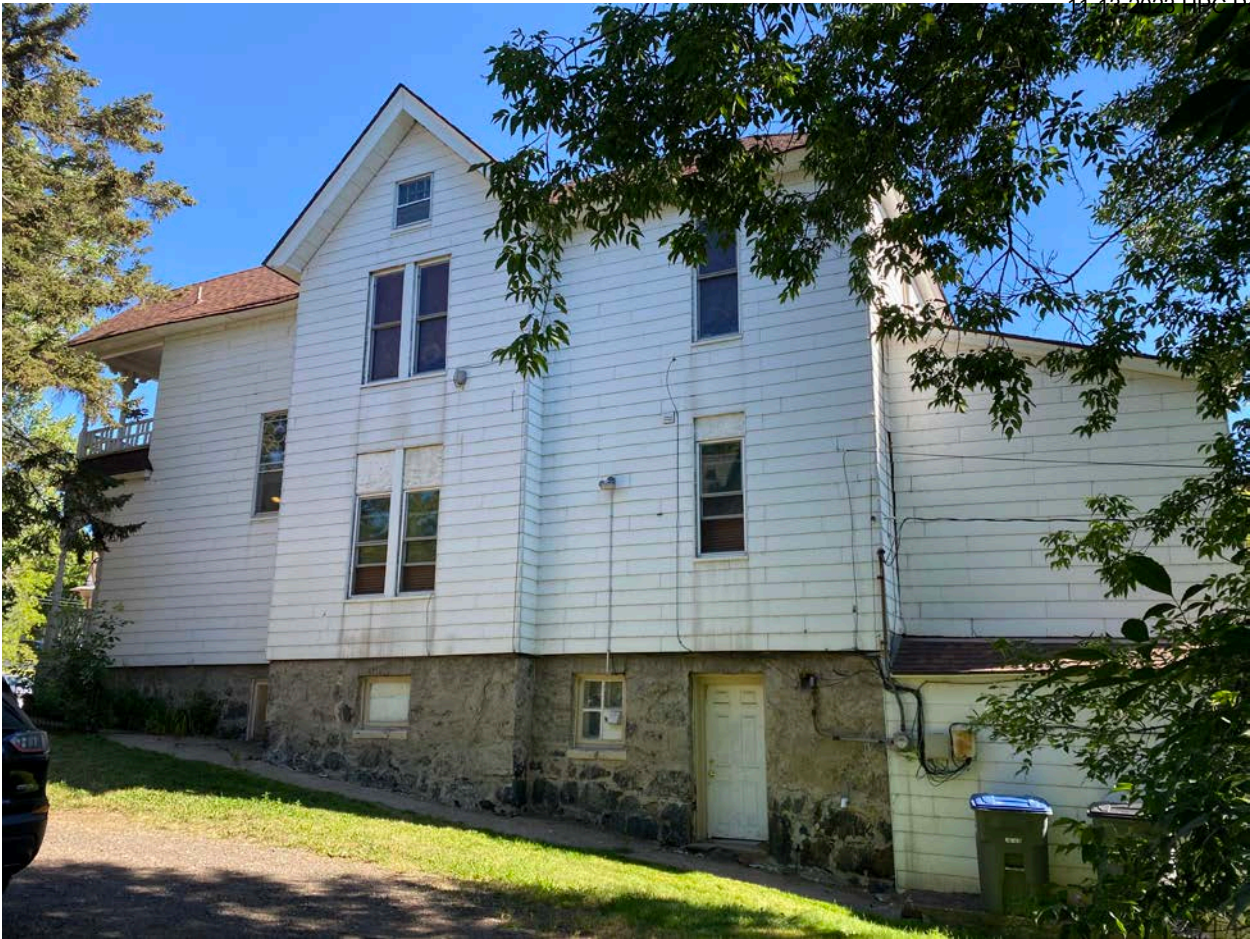
Photo 0007: View of west elevation, looking northeast.
