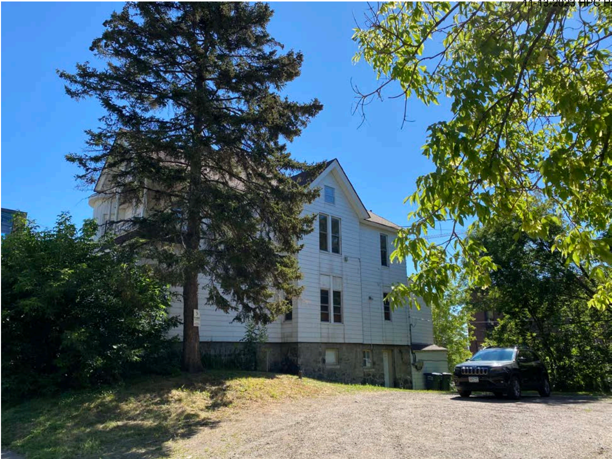
Photo 0008: View of west elevation, looking southeast.
