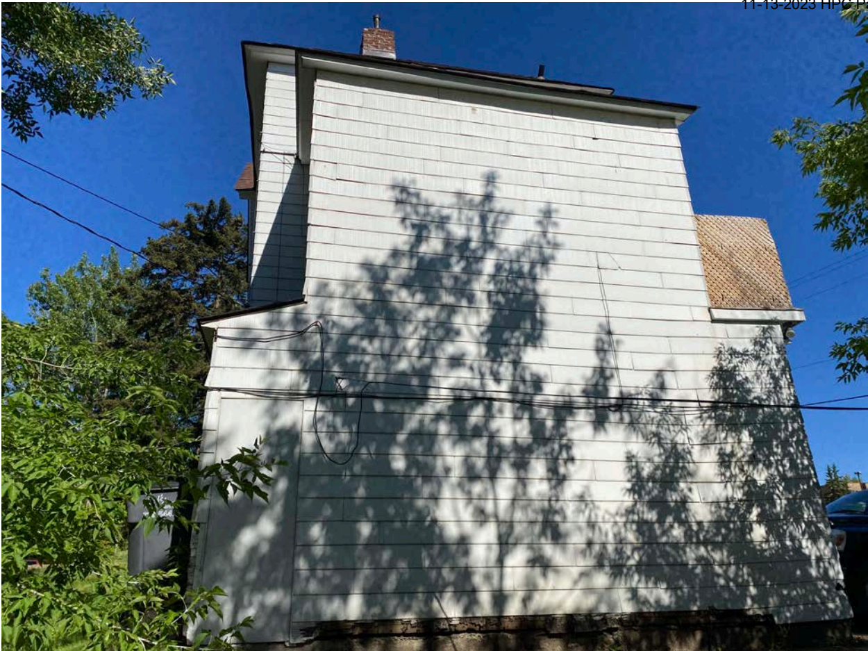
Photo 0006: View of south elevation, looking northeast.
