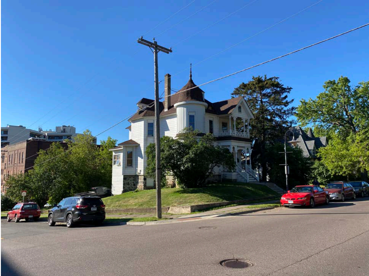
Photo 0001: View of north and east elevations, looking southwest.
