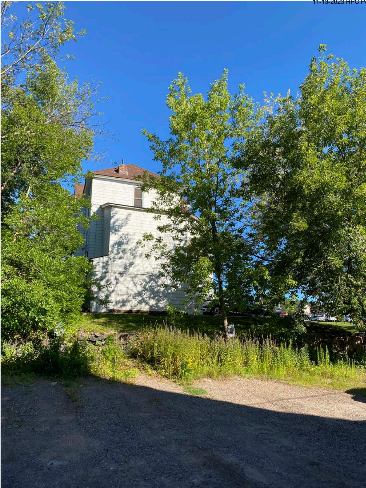
Photo 0005: View of south elevation, looking northeast.
