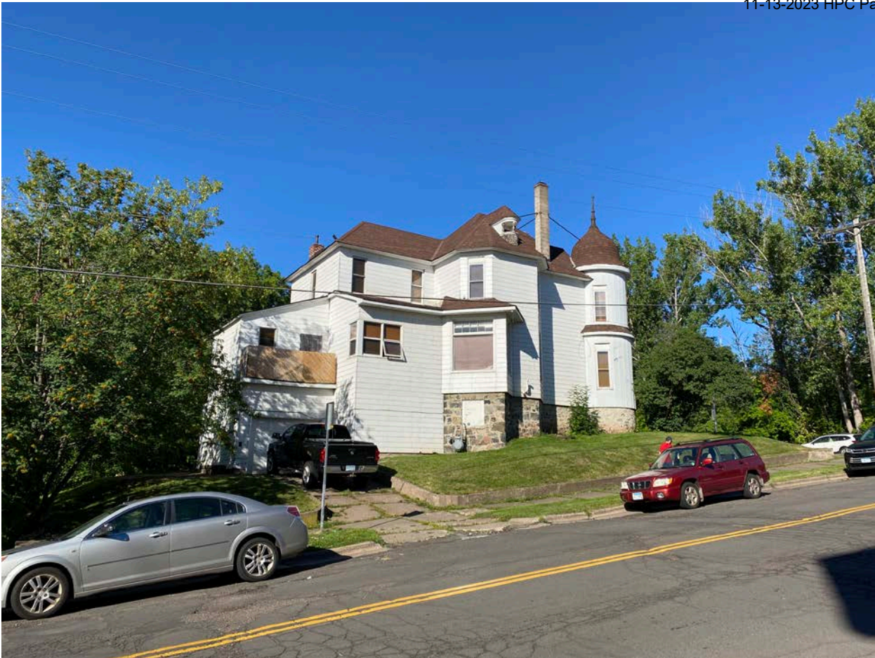
Photo 0004: View of east elevation, looking northwest.
