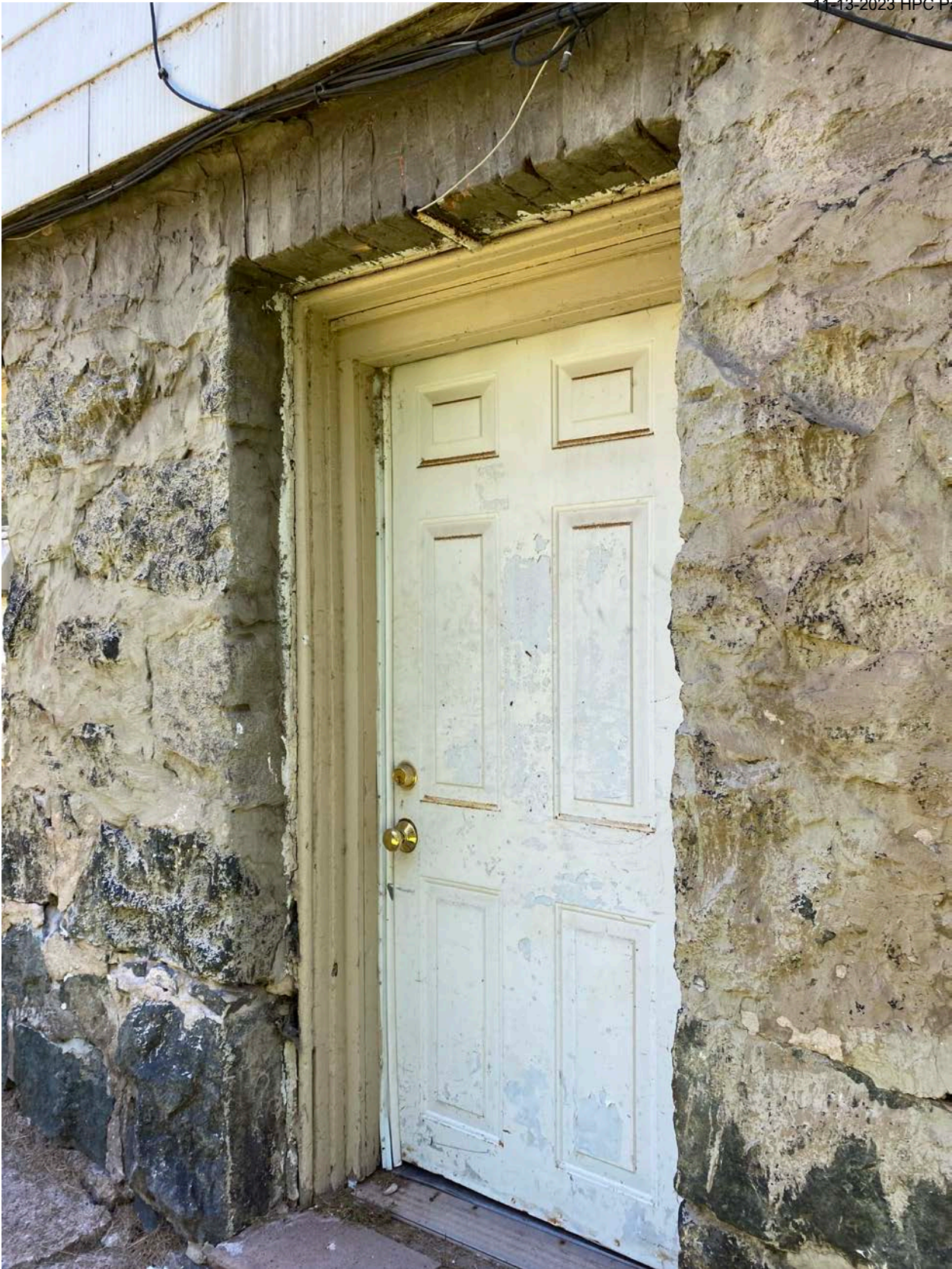
Photo 0012: View of entrance at west elevation, looking northeast.
