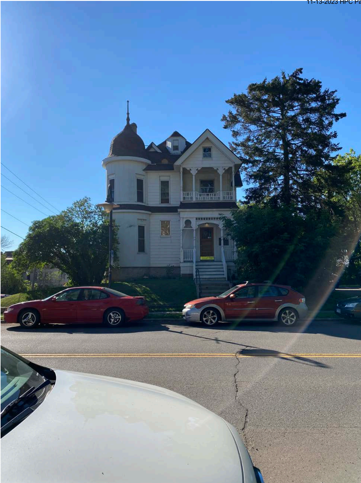
Photo 0002: View of north elevation, looking south.
