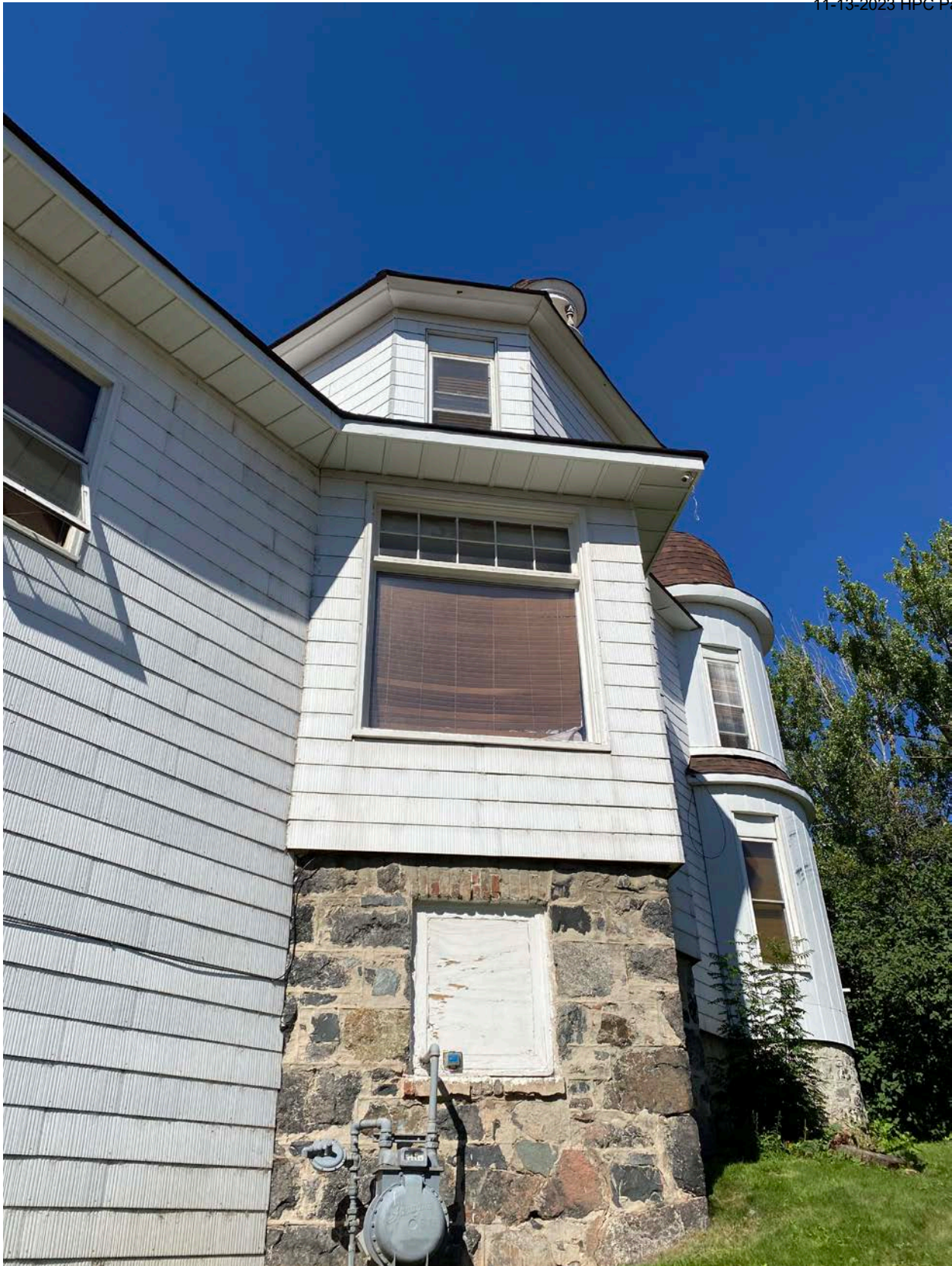
Photo 0016: View of east elevation, looking northwest.
