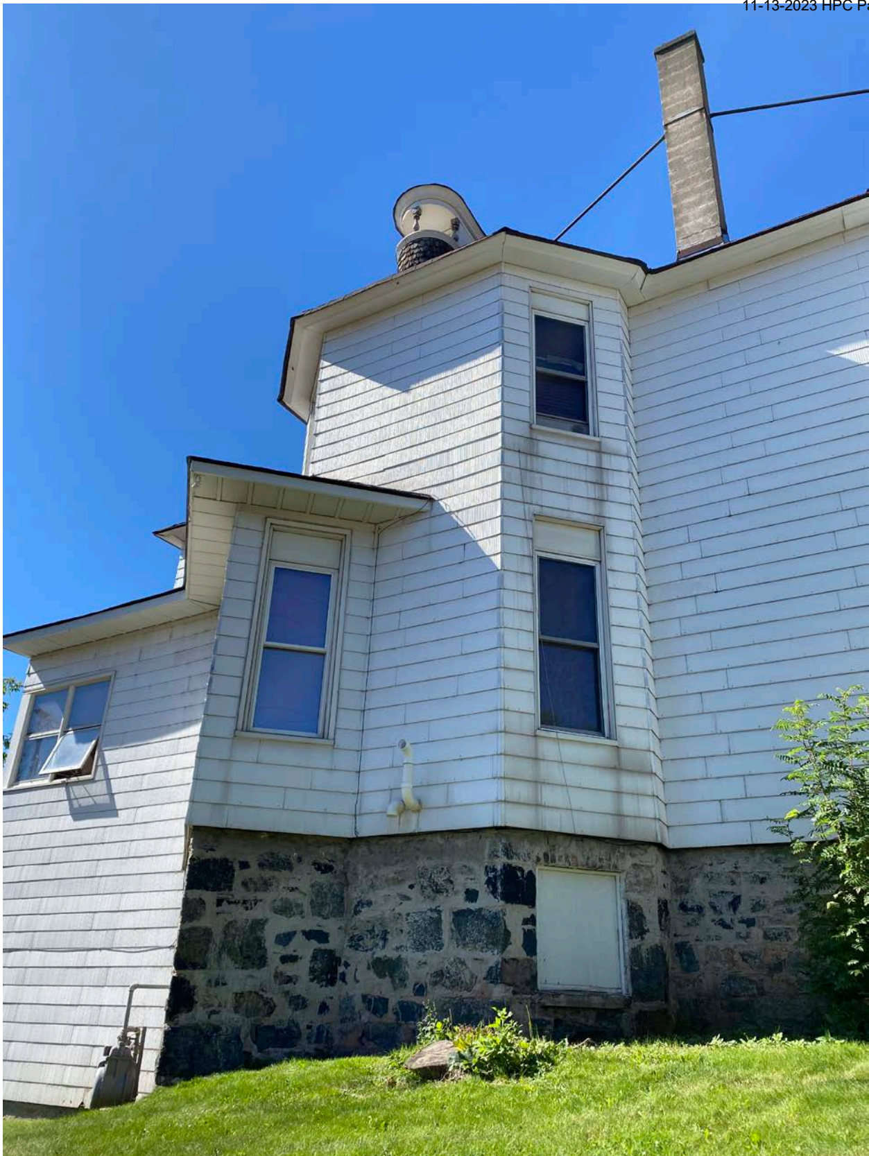
Photo 0017: View of east elevation, looking southwest.
