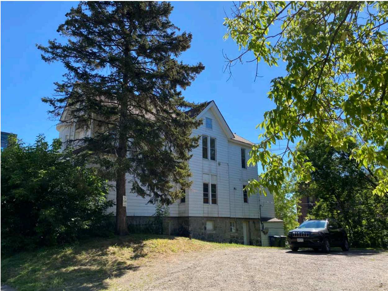
Photo 0008: View of west elevation, looking southeast.
