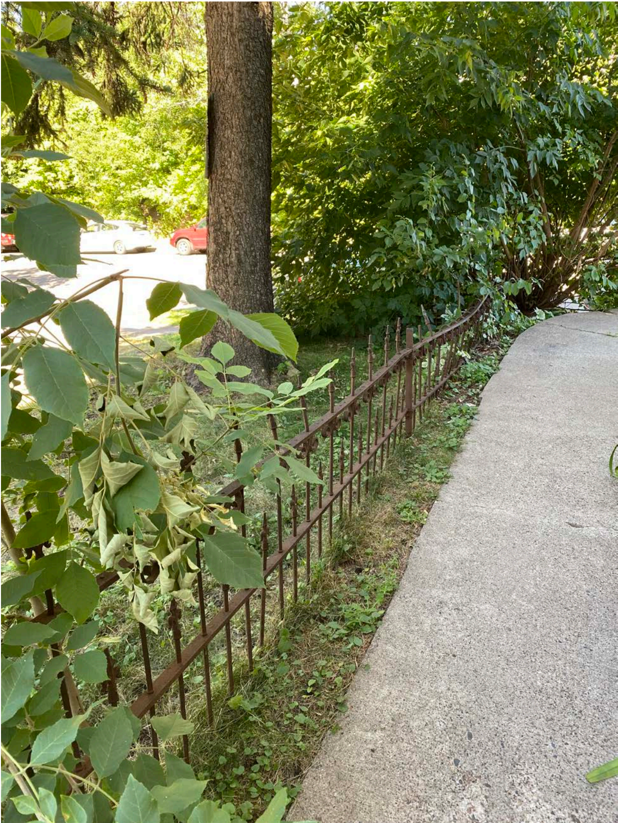
Photo 0010: View of metal fence at west elevation, looking north.
