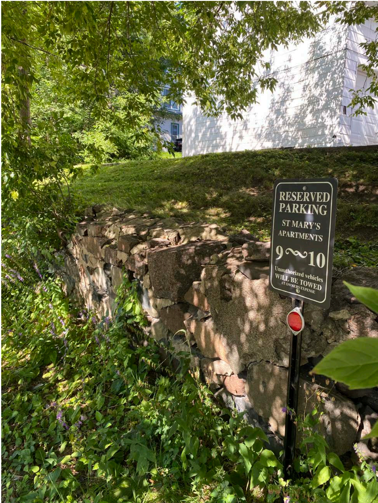
Photo 0013: View of stone wall to the south of the property, looking northwest.
