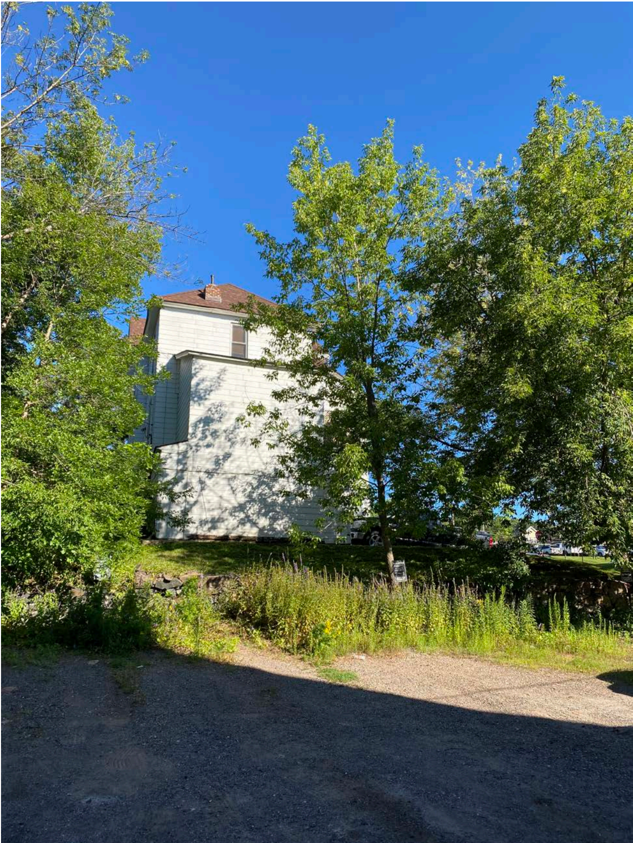
Photo 0005: View of south elevation, looking northeast.
