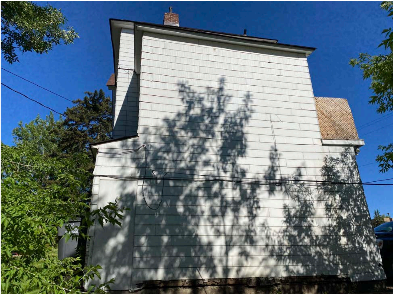
Photo 0006: View of south elevation, looking northeast.
