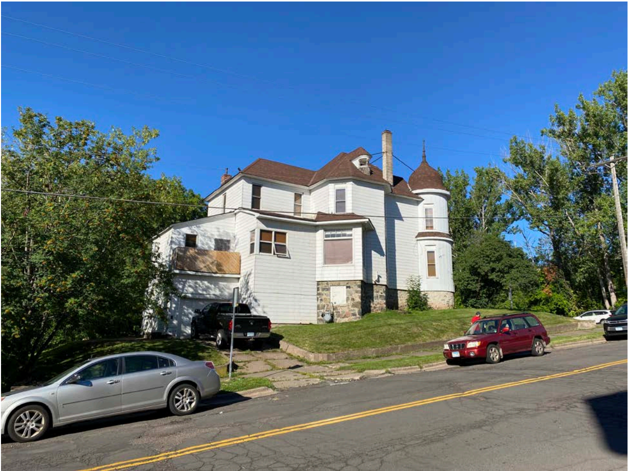
Photo 0004: View of east elevation, looking northwest.
