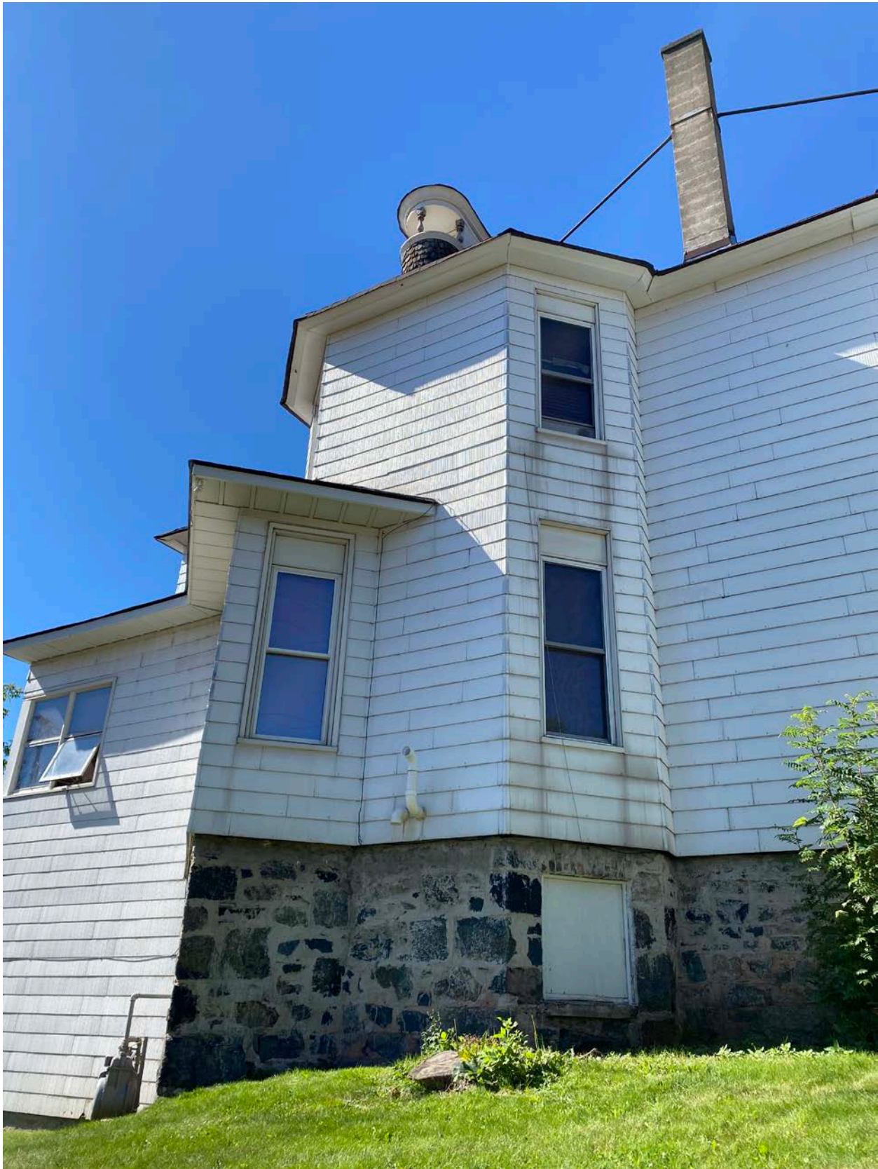
Photo 0017: View of east elevation, looking southwest.
