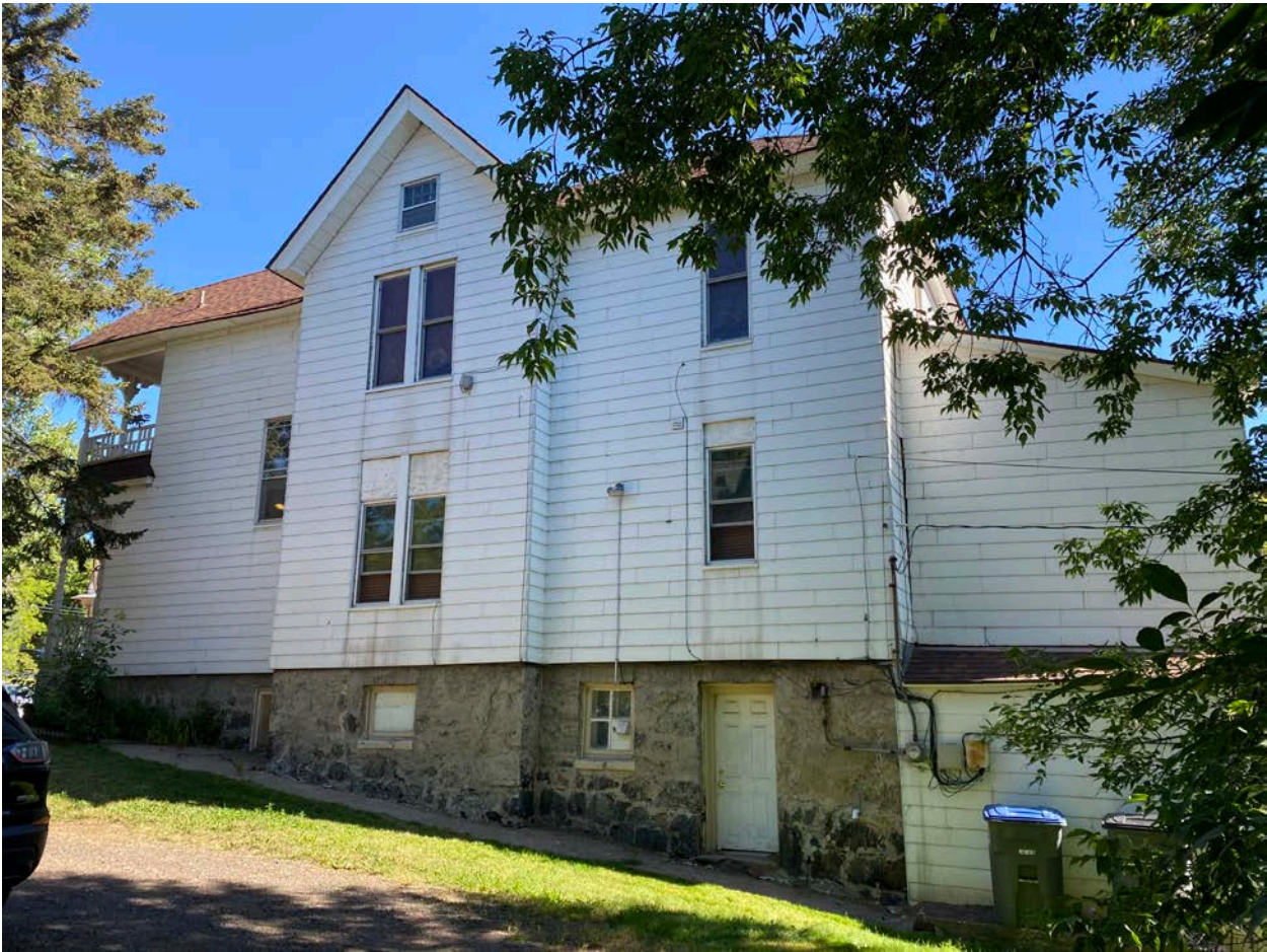
Photo 0007: View of west elevation, looking northeast.
