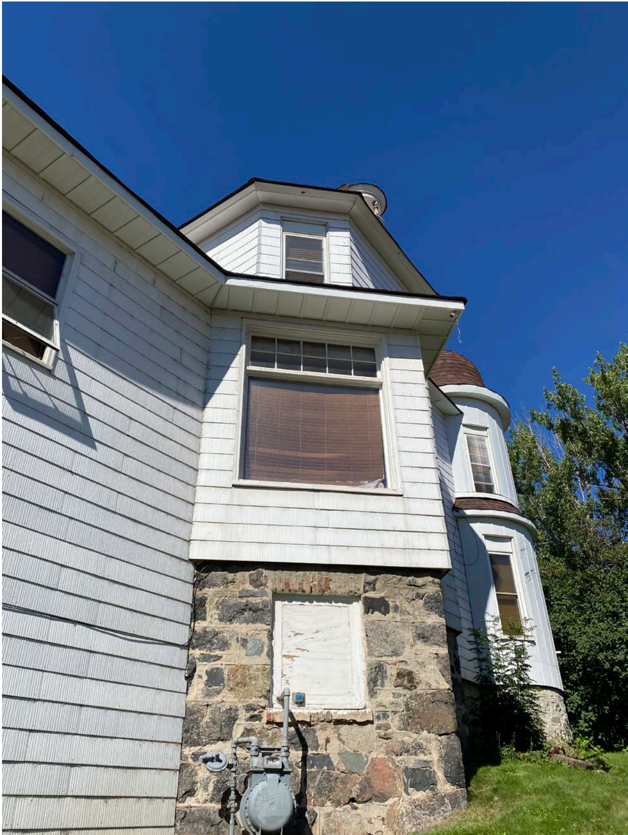
Photo 0016: View of east elevation, looking northwest.
