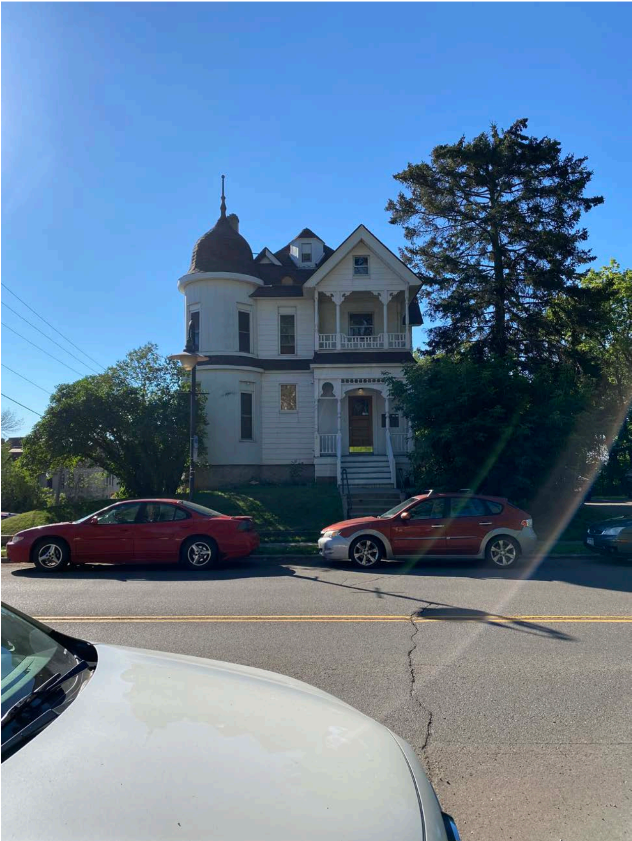
Photo 0002: View of north elevation, looking south.
