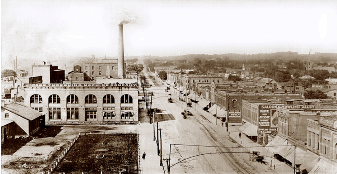
Turn-of-the-century photograph looking north along North Front Street. The three-story Stahl Hotel (1893) can be seen (with the corner awning) just to the upper right of center.
