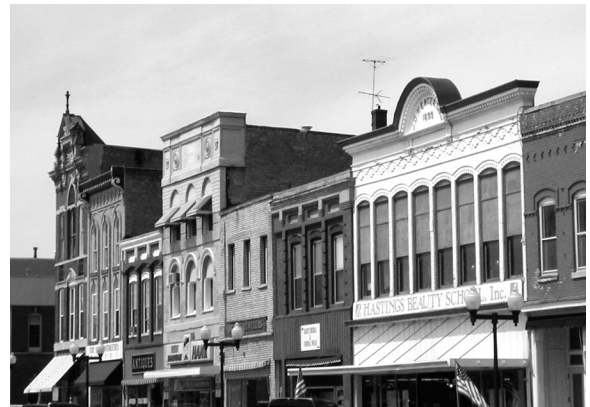
E. Second Street Historic District. Photo 2002.
