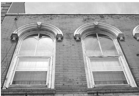
Elaborate window moldings are part of many nineteenth-century commercial facades.
