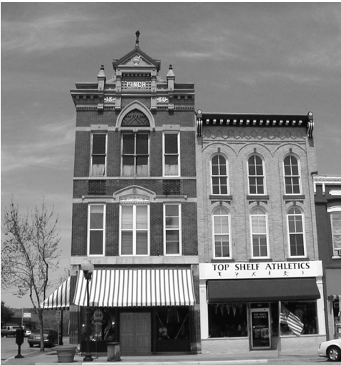
Red and cream brick as well as buff-colored limestone were used for commercial building construction. Unpainted brick and stone surfaces should not be painted.
