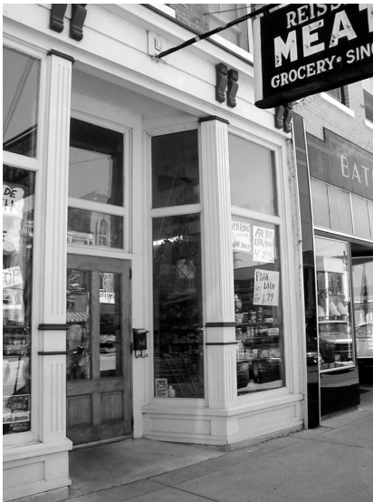
The renovation of this storefront included replication of many missing original features, including double-leaf doors, transoms, and fluted woodencolumns framing the display windows.
