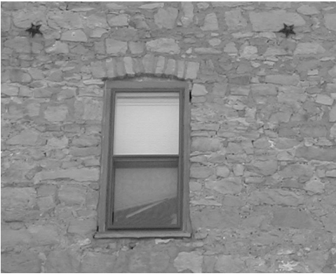
Historic features such as these masonry anchors should be conserved, as well as the limestone wall.
