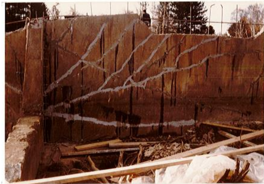
#11 10/16/85 FACE OF SOUTH WALL AFTER INJECTION
