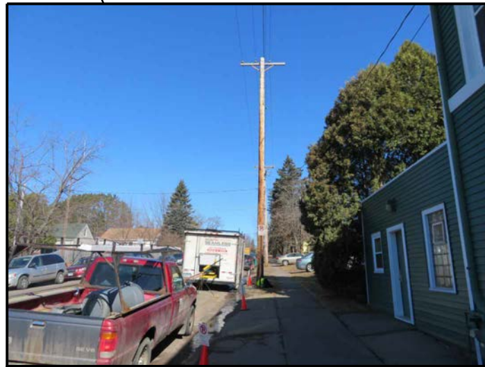
B SITE OVERVIEW [LOOKING NORTHWEST]
