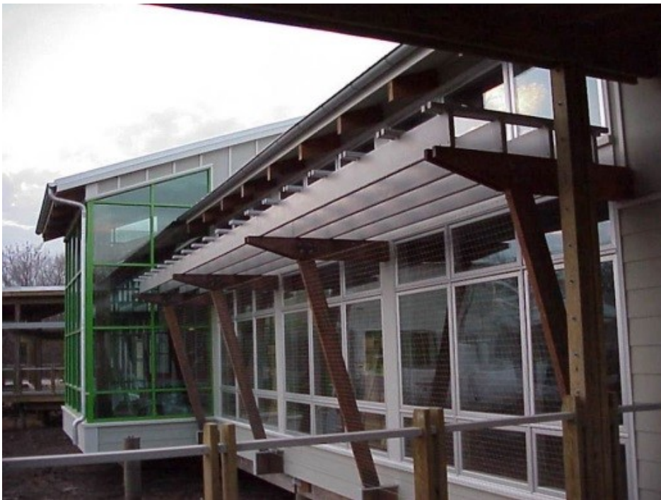
Netting installed on slanted wooden beams. Photo by USFWS.
