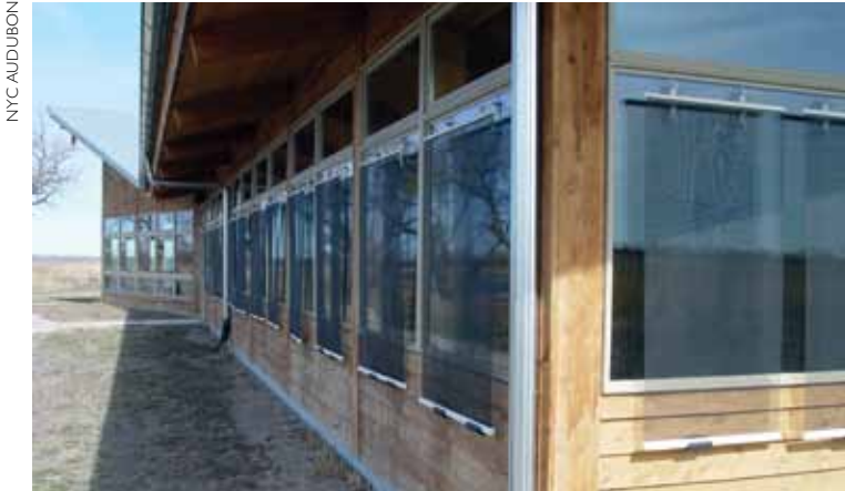
Window screening by Birdscreen installed at Rowe Audubon Sanctuary in Nebraska
