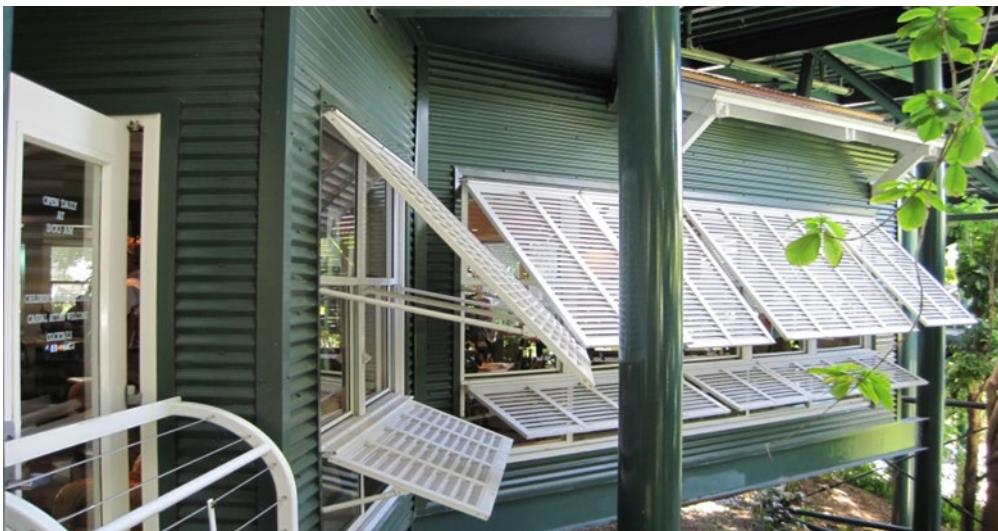
Shutters overhang windows at a facility at the San Diego Zoo. Photo by Christine Sheppard, ABC.
