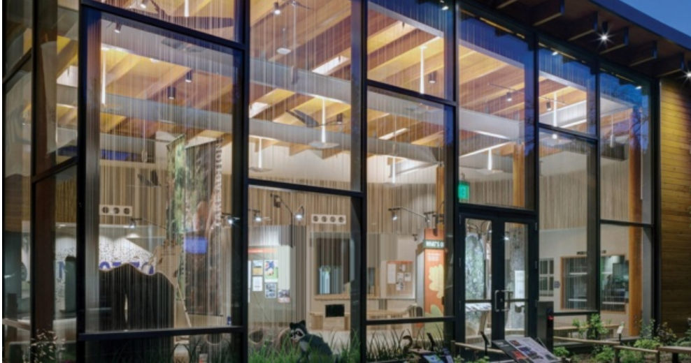
Etched, patterned glass provides a visual barrier to birds. Photo from https://www.walkerglass.com
