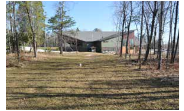
Chalet from staging area.
