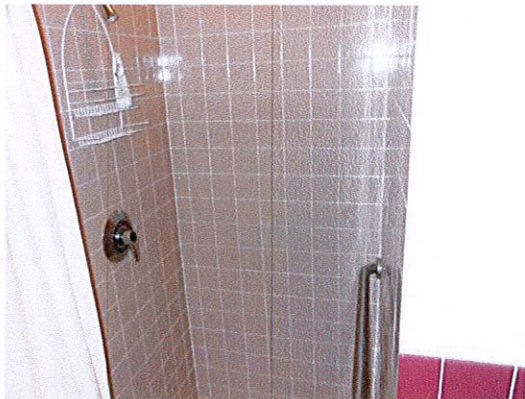
Photo 4: Add a shower seat, hand held shower wand and correct grab bars to create an accessible transfer shower.
