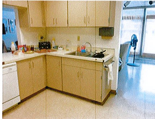
Photo 2: View of kitchen. There are currently no features of accessibility provided.
