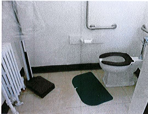
Photo 4: There are 2 single user toilet rooms on the main level.
