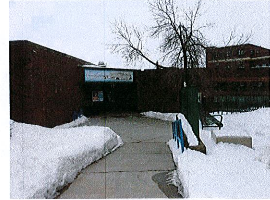
Photo 3: Reconstruct (or remove) the west route to the upper level entry. The slope is currently 15.5% for a distance of approximately 15'.
