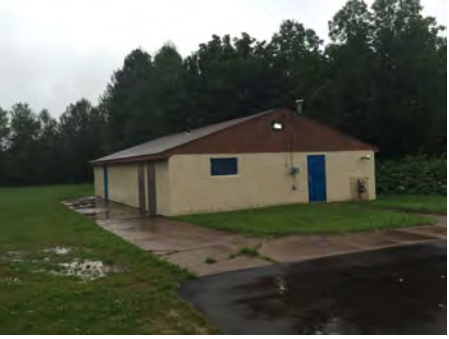
The existing building is no longer utilized
