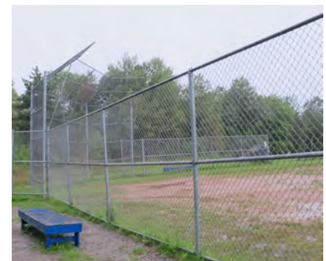
The softball field currently lacks dugouts
