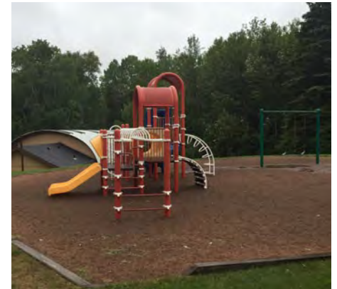
The existing playground is in fair condition
