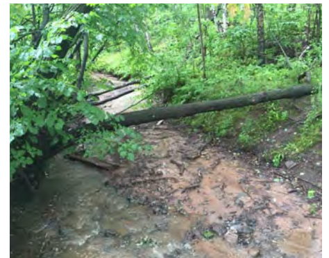
Erosion issues along 82nd Ave W Creek in the park
