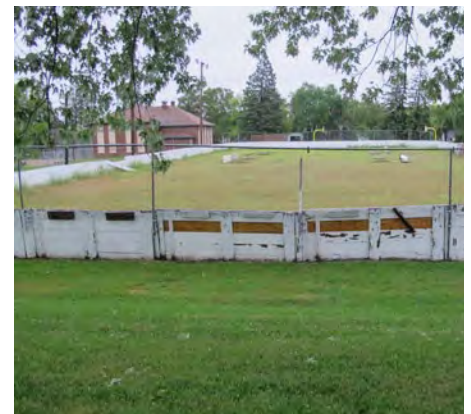
Boards at the existing broomball rink are in fair condition
