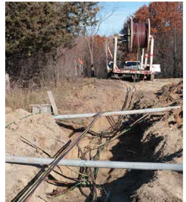
A water hydrant and electric pedestal stand along the new 5km snowmaking loop at Hyland Park in the Twin Cities. Below, excavation for buried snowmaking power.
