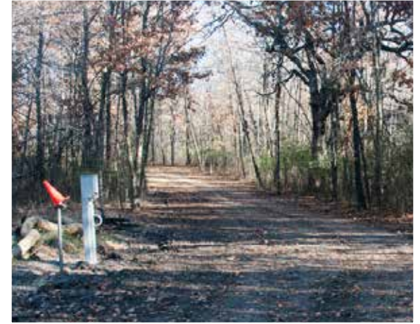
A water hydrant and electric pedestal stand along the new 5km snowmaking loop at Hyland Park in the Twin Cities. Below, excavation for buried snowmaking power.
