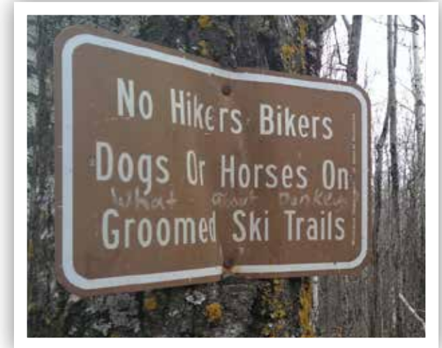
A sign at Lester Park needing to be replaced.
