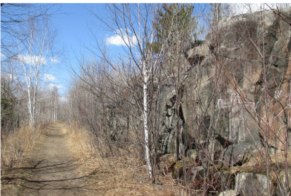
>>Photo Credit: Rock Cut, Barr Engineering
