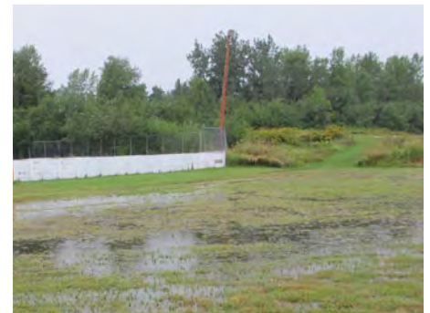
Poor stormwater management results in saturated conditions and unusable space
