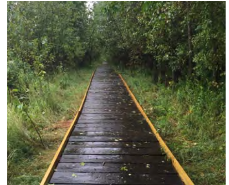
Most segments of the existing boardwalk have edges to improve wheelchair safety along the trail
