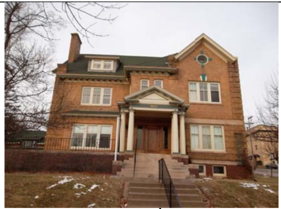
1831 East 3 rd Street
