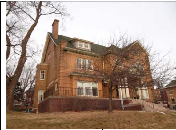
1831 East 3 rd Street
