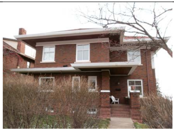
1902 East 3 rd Street
