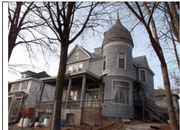
1523 East 3 rd Street
