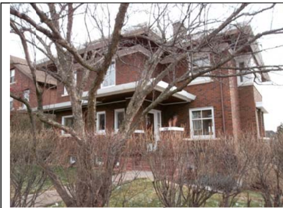
1902 East 3 rd Street
