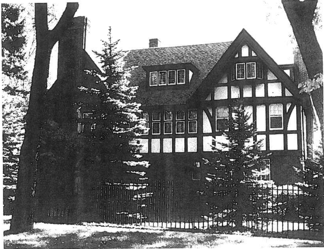
2314 East Fifth Street
