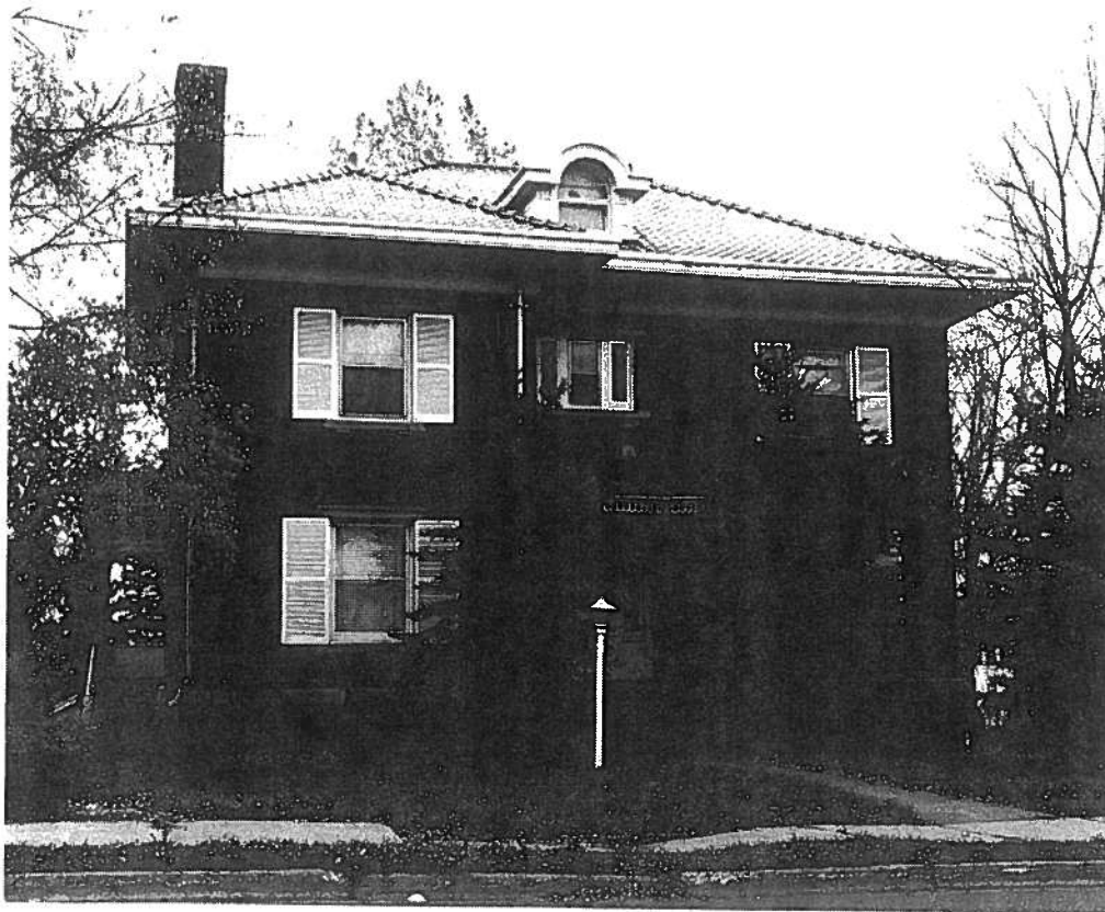
2020 East 3rd Street
