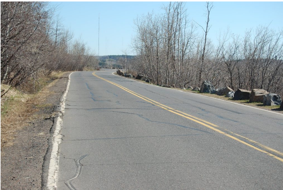
Figure 39. Western Extension from Overlook, Facing E
