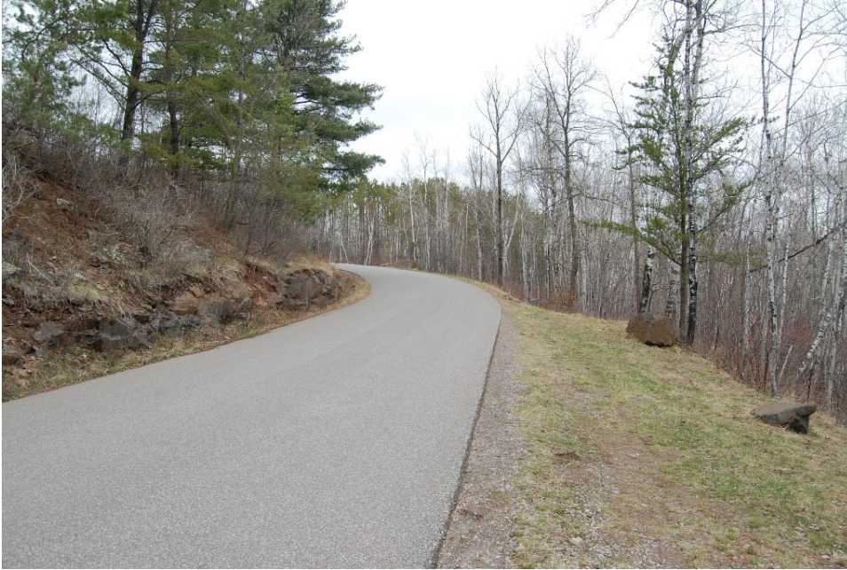
Figure 6. Seven Bridge Road, Facing S
