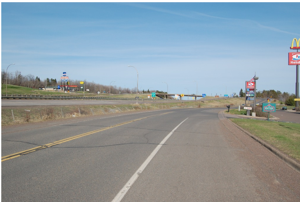
Figure 45. Parkway segment near I-35, Facing E
