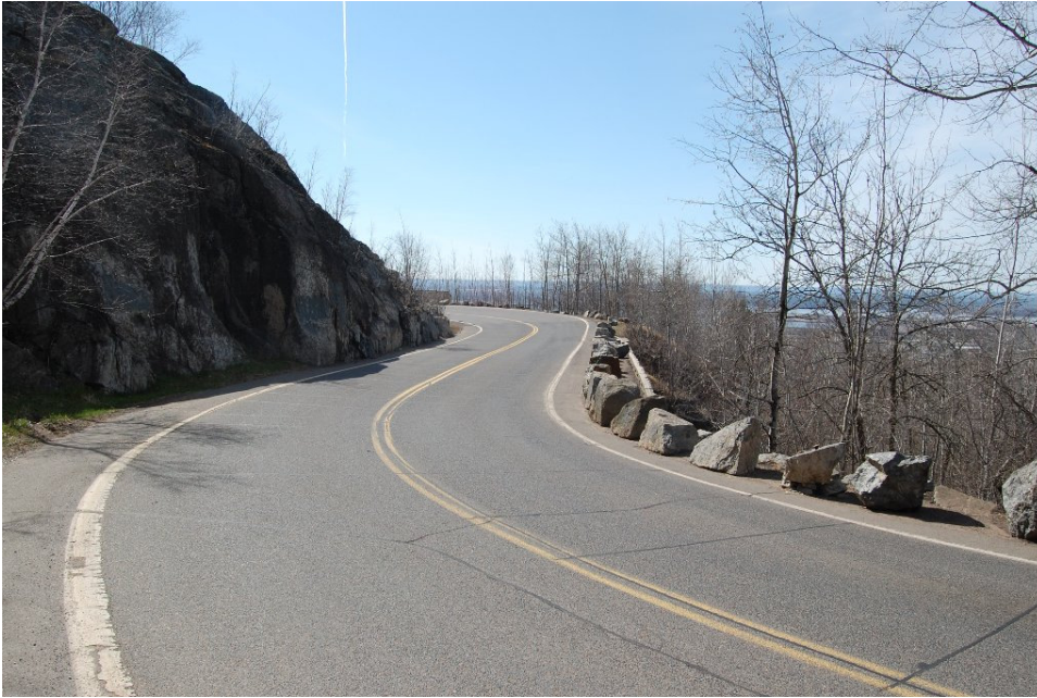
Figure 40. Western Extension from Culvert, Facing E
