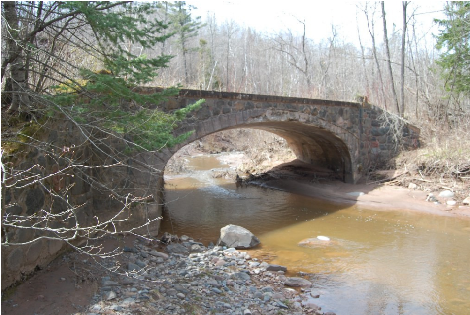
Figure 51. Bridge L6002, Typical Mission Creek Concrete Arch Bridge
