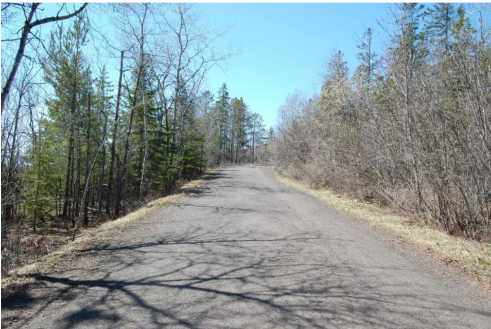
Figure 12. Hawk Ridge Roadway, Facing SW
