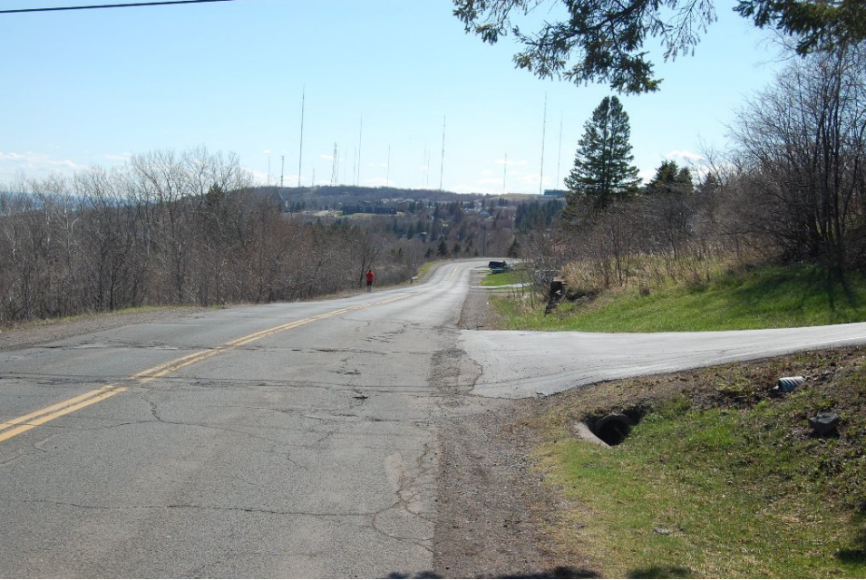
Figure 26. Rogers Parkway, west of Chester Creek, Facing W
