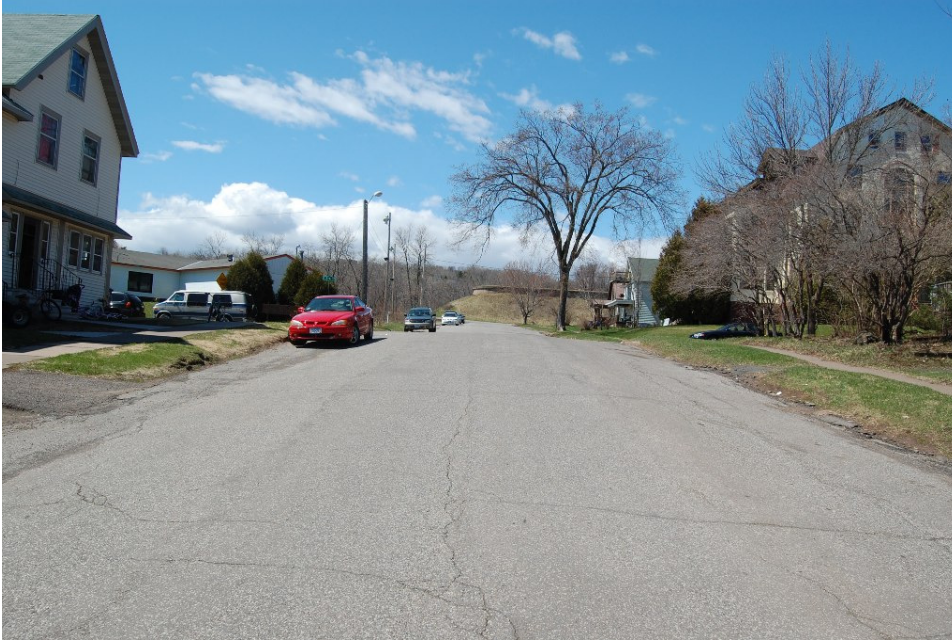
Figure 24. Chester Park Drive (N. 15th Ave. E.) from E. 5th Street, Facing NE
