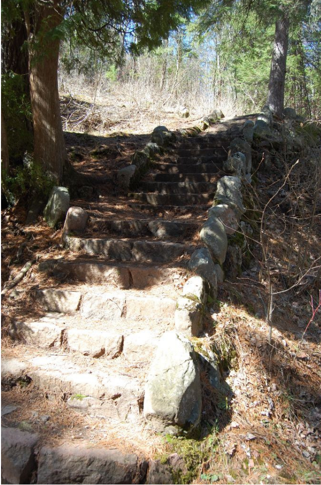
Figure 20. Congdon Park Drive, stone steps along pedestrian trail
