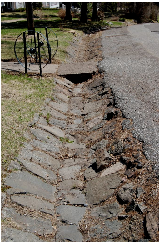
Figure 25. Stone gutter segment near Kent Road
