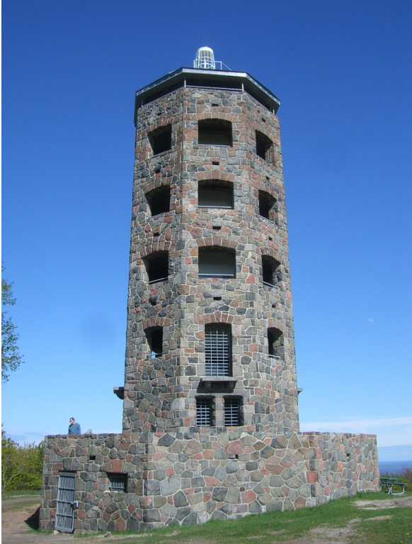
Figure 31. Enger Memorial Tower, Facing S
