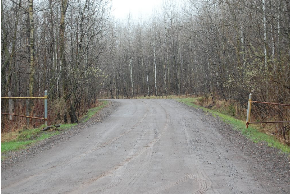
Figure 48. Parkway from N. 80th Ave W.
