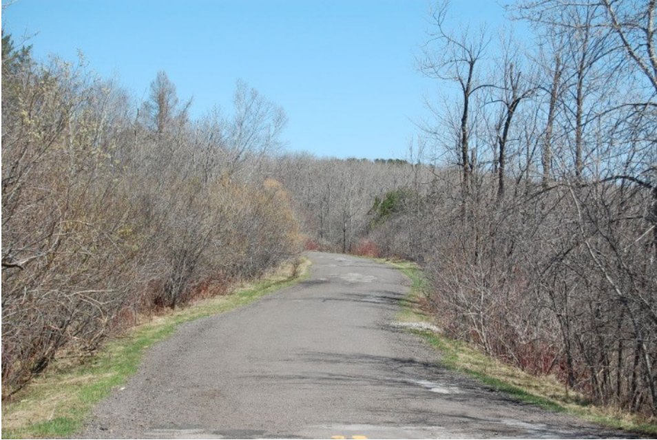
Figure 11. Hawk Ridge Roadway from West Overlook, Facing NE
