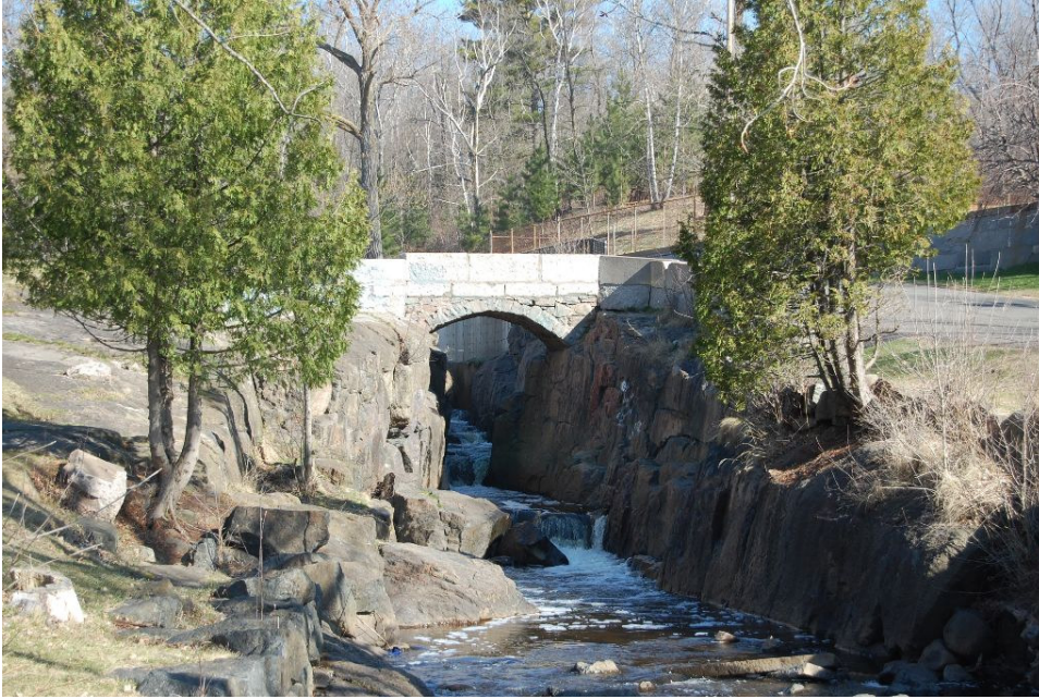
Figure 36. Stone Arch Pedestrian Bridge, Facing N
