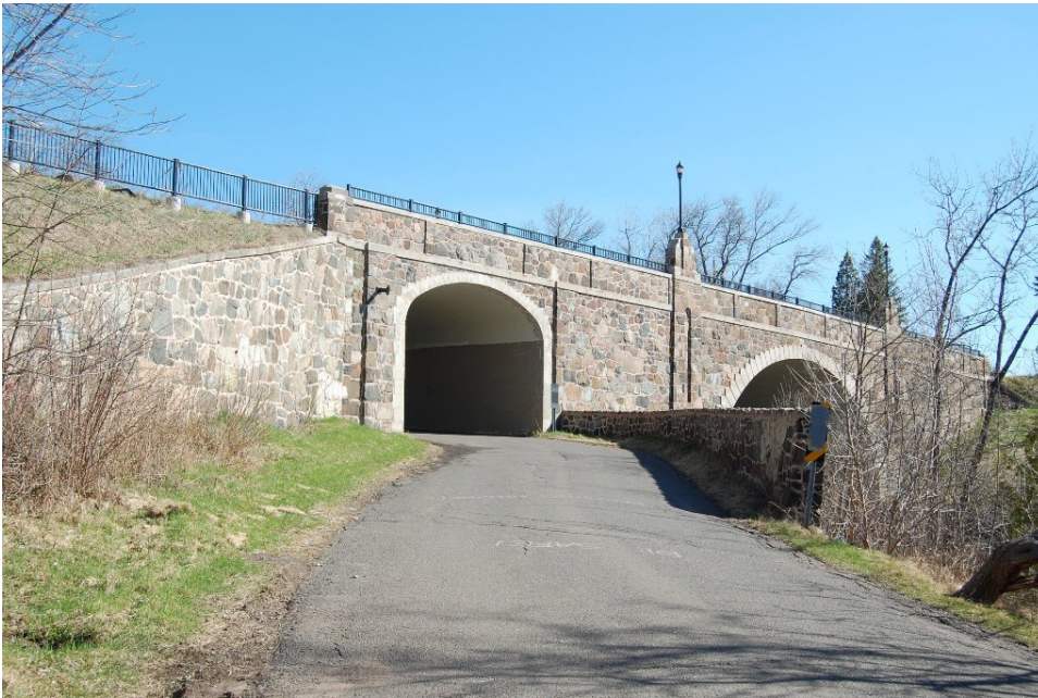
Figure 35. Lincoln Park Bridge (L-8477), Facing NE
