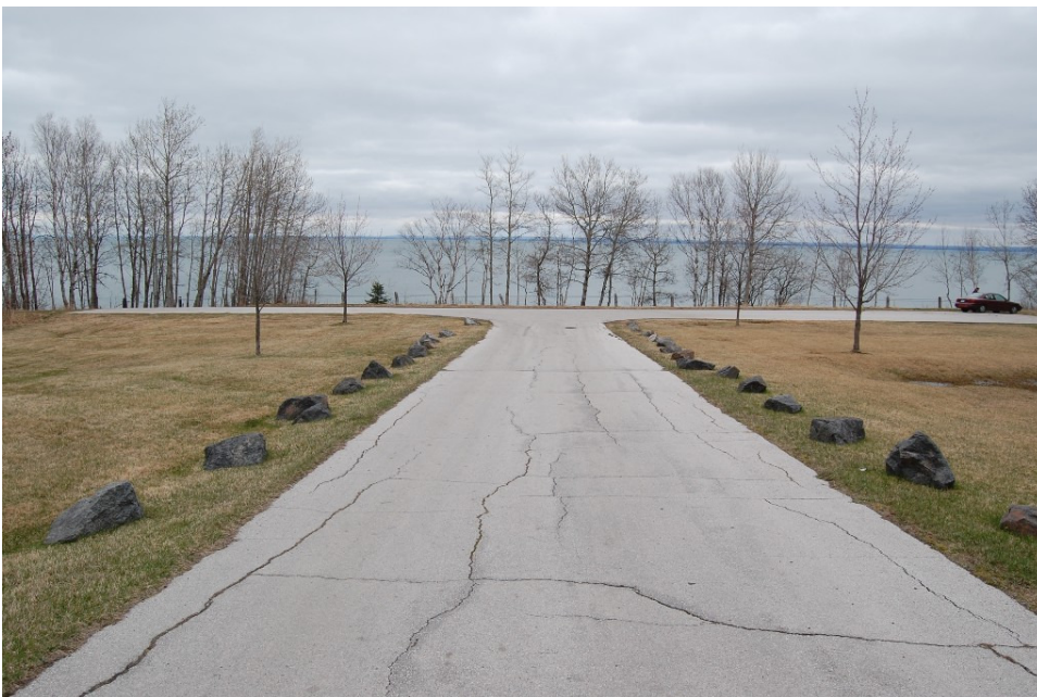
Figure 2. Typical T-shape pullout at 7002 Congdon Boulevard, Facing SE
