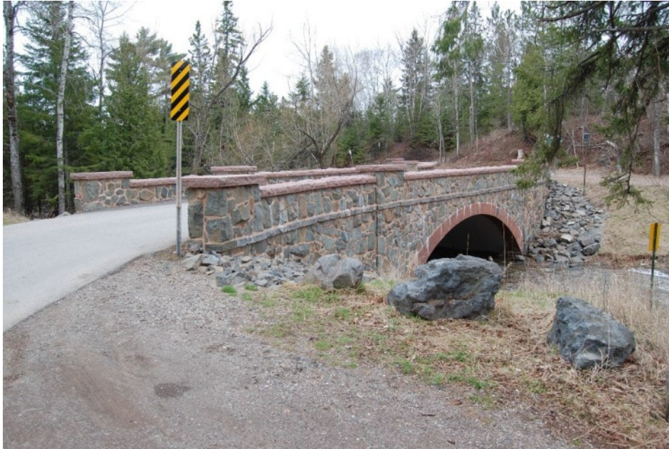
Figure 8. Bridge 69671 (2007), typical replacement bridge, Facing SW
