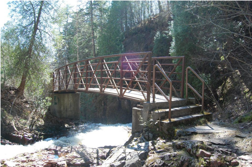
Figure 21. Congdon Park Drive, example of modern pedestrian bridge crossing creek
