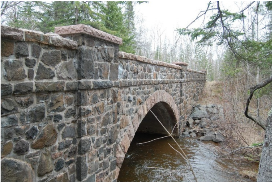
Figure 7. Bridge L8505 (c.1912), typical original bridge, Facing SE
