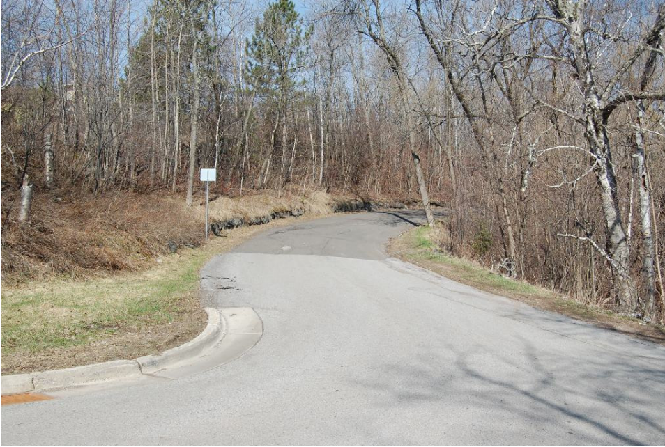
Figure 34. Lincoln Park Drive, From W. 10th Street, Facing N
