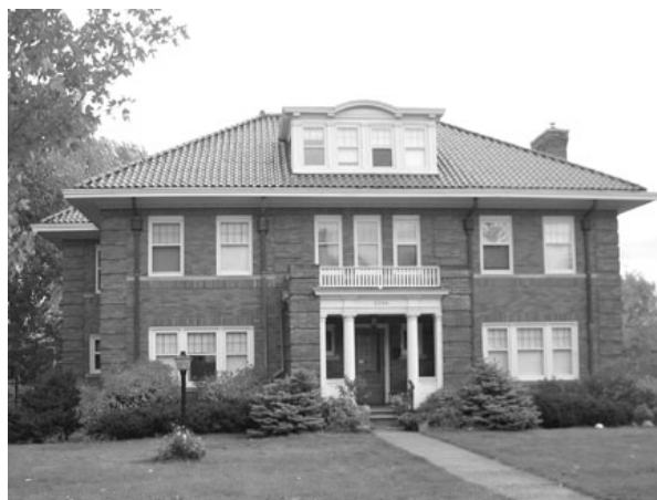
This 1924 house displays brick quoining at the corners, a typical element of the Classical Revival style. The house is located at 2304 East Third Street and was first occupied by Carl and Emily Meeske.
