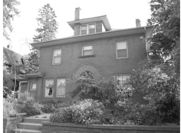
The Walter and Sarah Turle Residence at 2216 East Superior Street, built in 1899 and designed when Tenbusch was in partnership with I. Vernon Hill, it predated most of the houses in the East End and shows early Prairie School influences.
