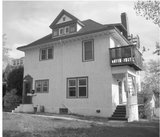
The Cullum House as it appears today without its corner tower and circular porch.
