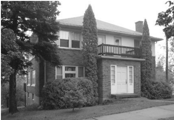
The Lorace and Florence Catterson Residence, 1923, is actually a duplex located at 2702-04 East First Street.
