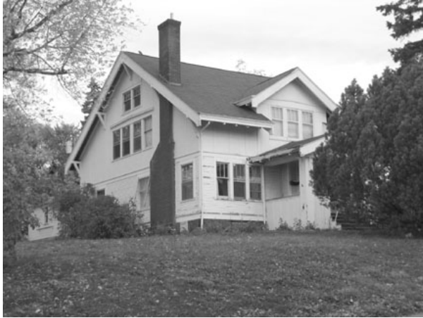
A modified Bungalow form is created by extending the gable roof only down to the half-story point. Craftsman details abound on this 1913 house at 2309 East Second Street.
