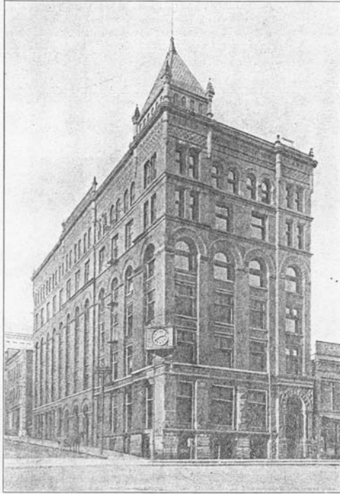
THE FIRST NATIONAL BANK BUILDING DULUTH, MINN.
