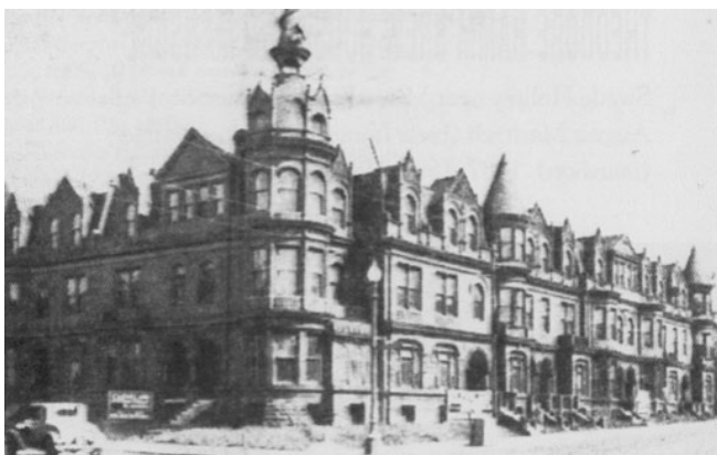
Hunt designed this elaborate “terrace” with eleven 3-story dwelling units in 1888 for a design competition. It was located on 17 th Street in south Minneapolis until its demolition in 1932.
