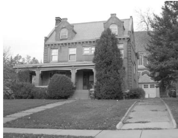
The Henry and Amy Fee House at 2305 East Third Street, 1906, architect unknown, incorporates Tudor masonry elements: parapet gable roofs and dormers.
