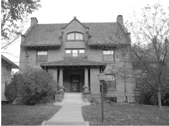
The William and Mary LaRue House at 2131 East Second Street, built in 1909, was one of only four truly Eclectic style houses in the neighborhood. Designed by William Hunt, it incorporates, a green glazed tile parapet gable roof (English), Tuscan columns, Roman brick, rusticated redstone foundation.
