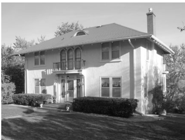
The James and Flora Harper House at 2502 East Superior Street, 1919, is one of the simpler Classical Revival houses, defined by its arched windows and classical ornamentation. It was designed by architect Arthur Hanford.
