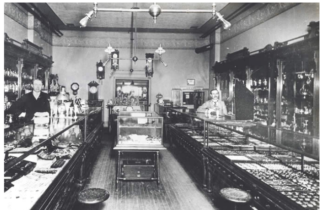
Early interior view of the Bagley & Co. shop. Photo courtesy of Bagley & Co. 79
