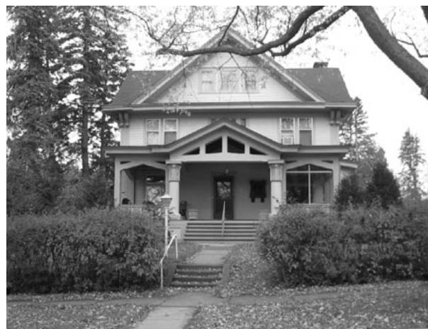
Another Bray & Nystrom house is the John and Alice Elliott Residence at 2429 East Second. It dates to 1908.
