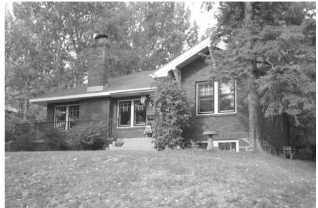
The Godfrey and Emma Westberg Residence at 2615 East Superior Street, 1926, is a fine example of a simple Craftsman style.
