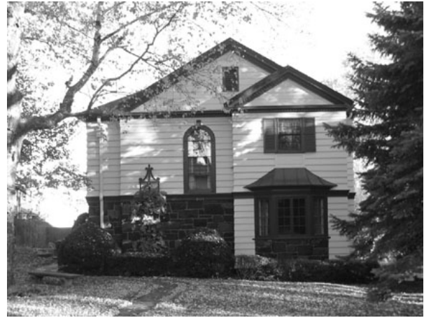
The second Cassius and Minnie Bagley House at 2424 East Second Street (the first was located behind this at 2431 East First Street) is a unique design by Starin dating to 1933.
