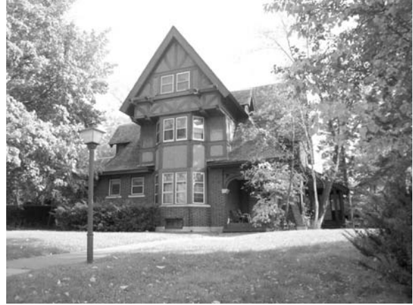
Hill's own home, 2220 East Superior Street, built the same year as the Crosby House, was designed in the English/Tudor Revival Style.
