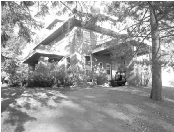
The Harvey and Elizatbeth Williamson House at 2400 East First Street, 1905, is an excellent example of the Prairie style. The architect is unknown.
