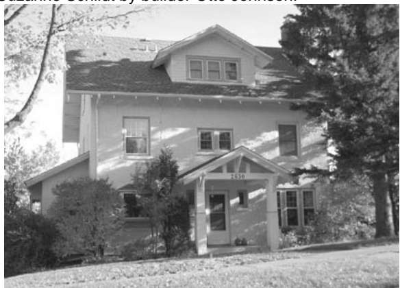
The Carl and Catherine Ehle House was built in 1912, architect unknown, and demonstrates how stucco was used in Craftsman houses.
