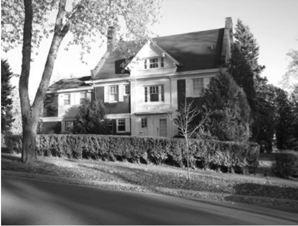
Puck designed the Richard and Neva Griggs Residence in an Eclectic style. It dates to 1906 and is located at 2502 East Second Street.
