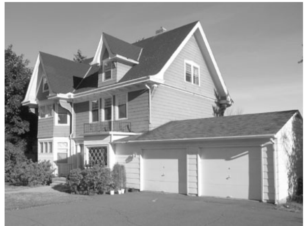
The Daniel and Alice Waite Residence at 2510 East Superior Street dates to 1904 and is credited to Wangenstein.
